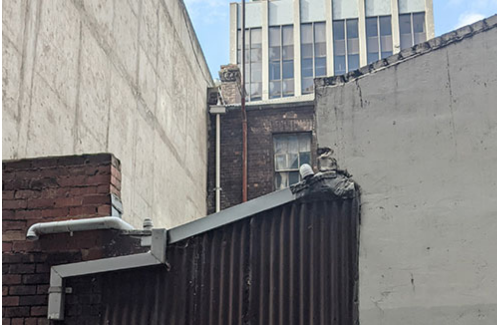
Chimney and intact rear brickwork clearly visible from the rear laneway
