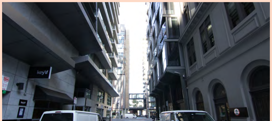
Figure 79 Enclosed projections over this laneway shift the perceived building alignment by projecting the full mass forward of adjacent heritage buildings.
