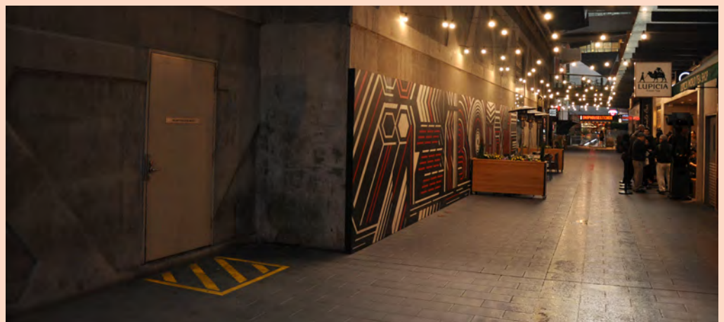
Figure 7 Steps in the building alignment or service doors can create entrapment spaces
