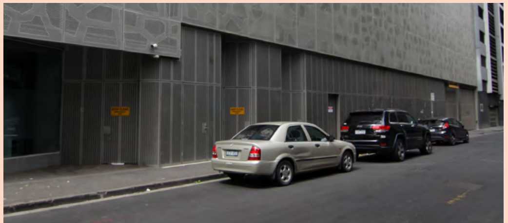
Figure 87 The use of perforated mesh abutting the public realm reduces the quality of this laneway within Southbank
