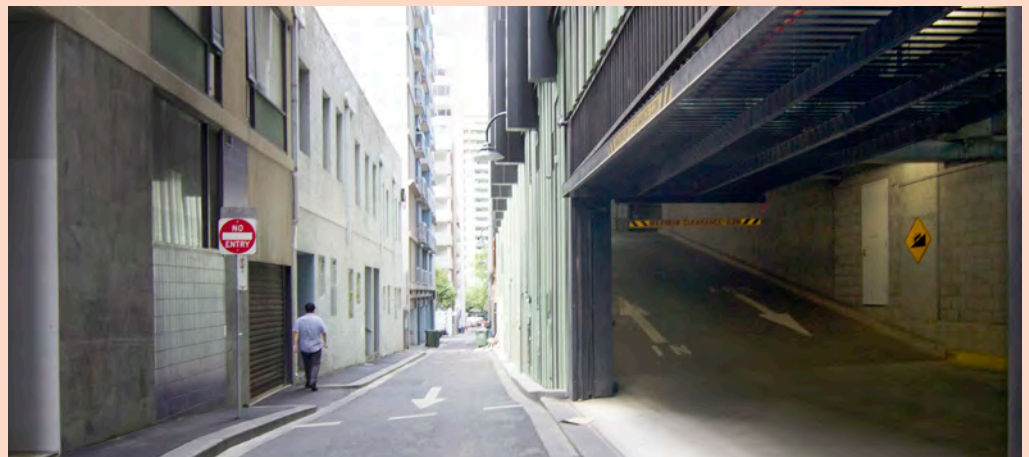
Figure 47 A carpark reliant on ramped floor plates is more difficult to adapt in the future.
