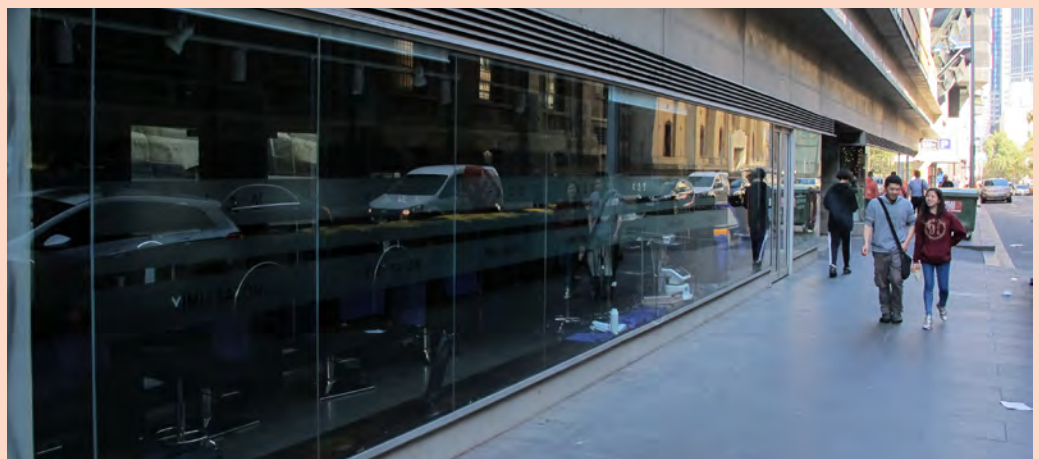
Figure 73 Long expanses of glass without pilasters or pronounced building entries result in a poor public realm interface lacking in rhythm, depth and tactility.
