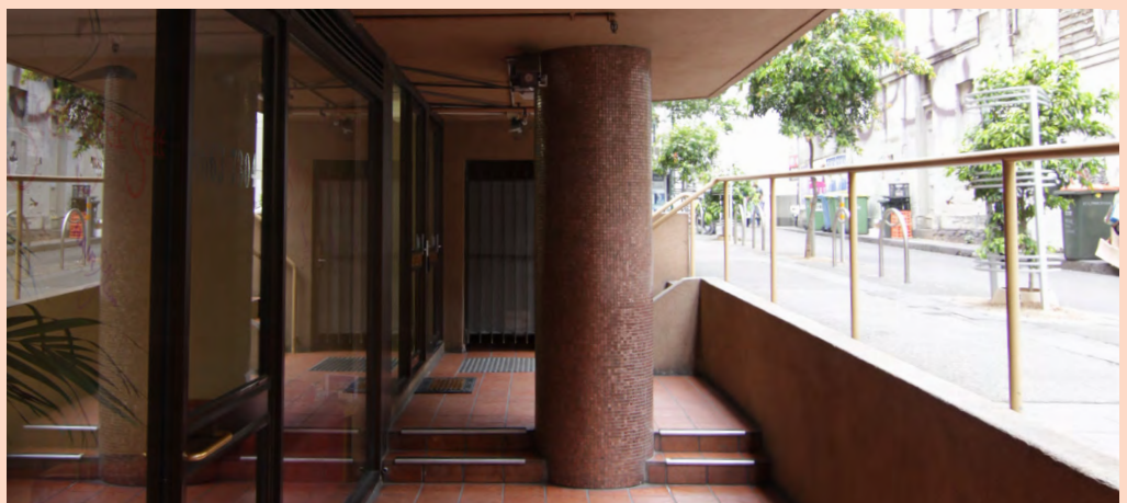
Figure 16 The depth of this colonnade and location below street level reduces the connection between building occupants and the street.
