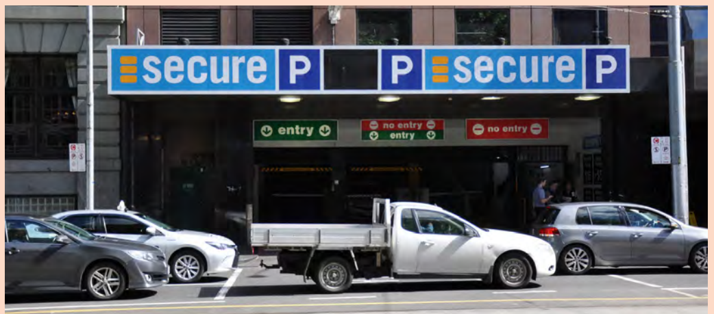
Figure 18 This carpark entry takes the full width of a main street building frontage, and significantly impacts upon the quality of the streetscape.
