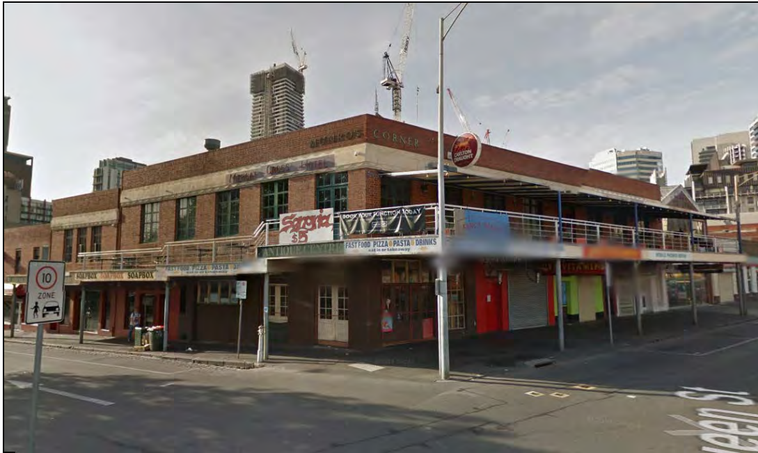
143-151 Therry Street, Melbourne - source: Street View
