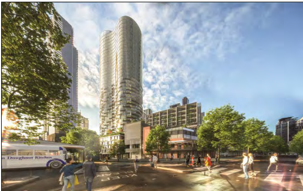
Munro Site Development looking south east from corner of Queen and Franklin Streets – source: Application documentation
