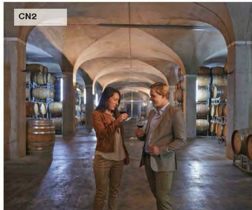
CN2 Vaults Exemplar Yering Station Basement // Off form concrete ceiling to vaulted retail tenancies subject to further design development resolution.
