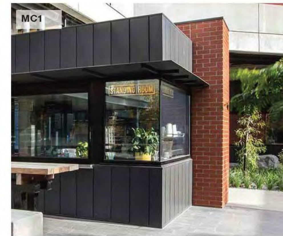
MC1 Metal Wall Cladding Exemplar Monash University, Monash Connect, Caulfield Campus // Six Degrees Architects
