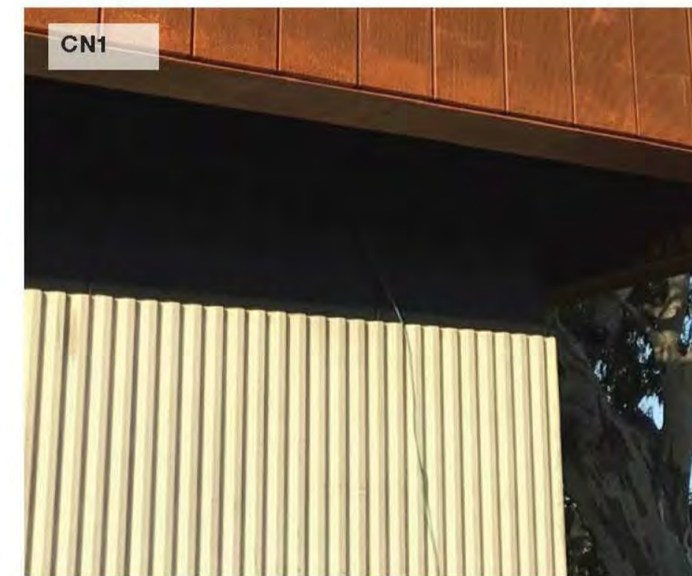
CN1 Concrete with Formliner Texture Victoria Police Mernda 24 hour Station // Six Degrees Architects
