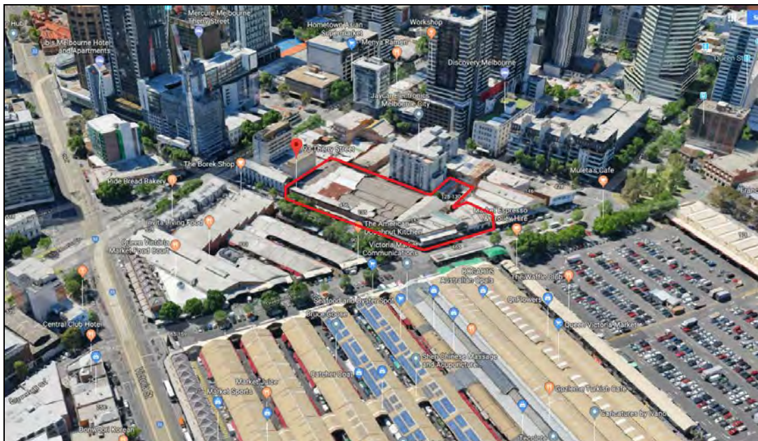
Aerial View of the site looking south-east – source: Google Maps 2017
