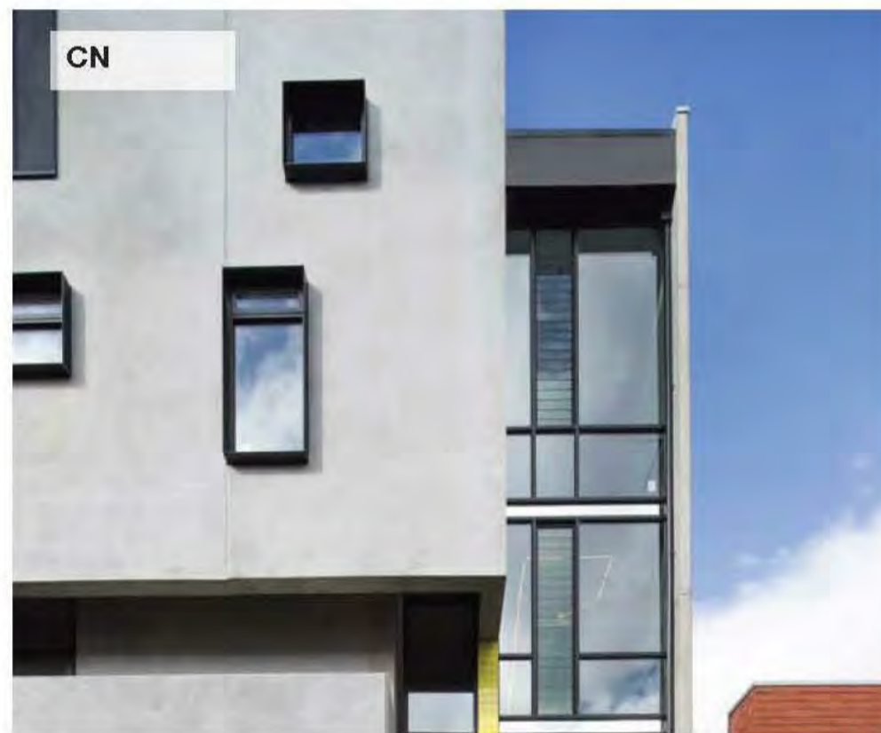
CN Precast Concrete Exemplar Class 2 Finish // 3-5 Jessie St, Cremorne // Six Degrees Architects
