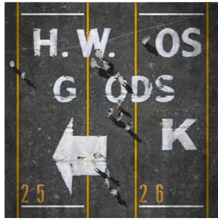
03 | ASPHALT WITH MARKINGS
