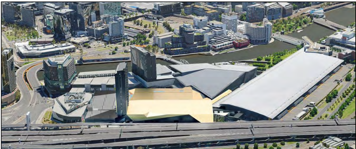
View of works from the south across the Freeway: Source: Application documentation
