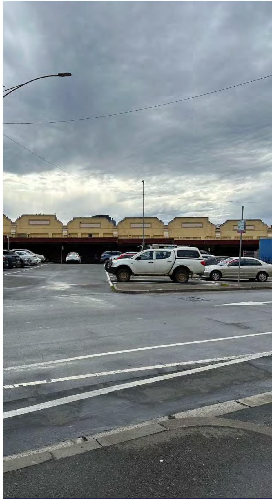
DPO11 Parcel D (future Tower 1) from Franklin Street
