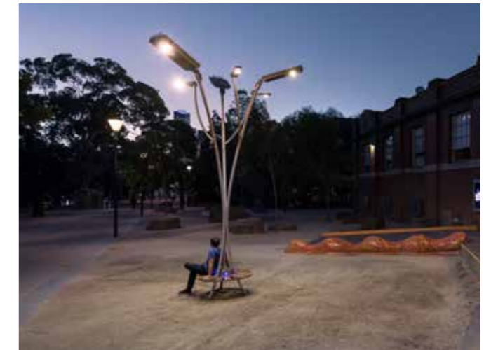
Multi-functional lighting installations
