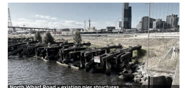
North Wharf Road - existing pier structures
