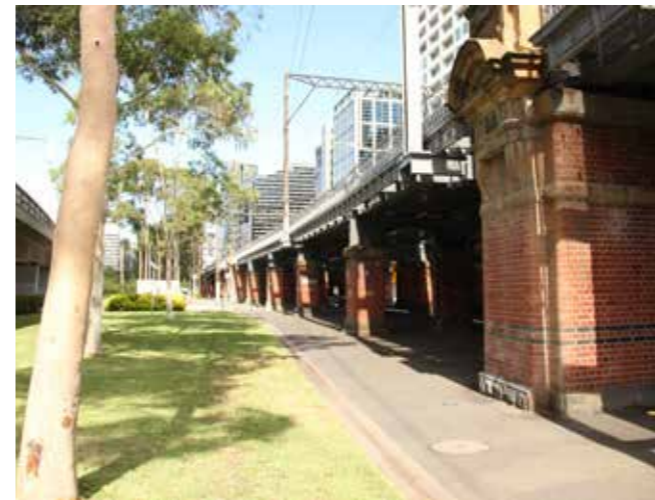
Railway viaducts - Flinders Street
