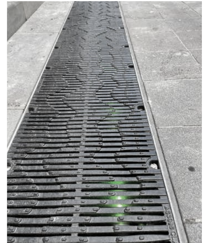
Custom grates designed to reduce litter entering waterways
