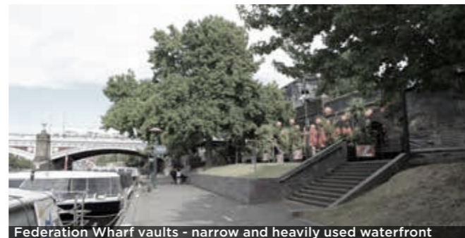
Federation Wharf vaults - narrow and heavily used waterfront
