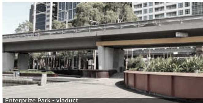
Enterprize Park - viaduct
