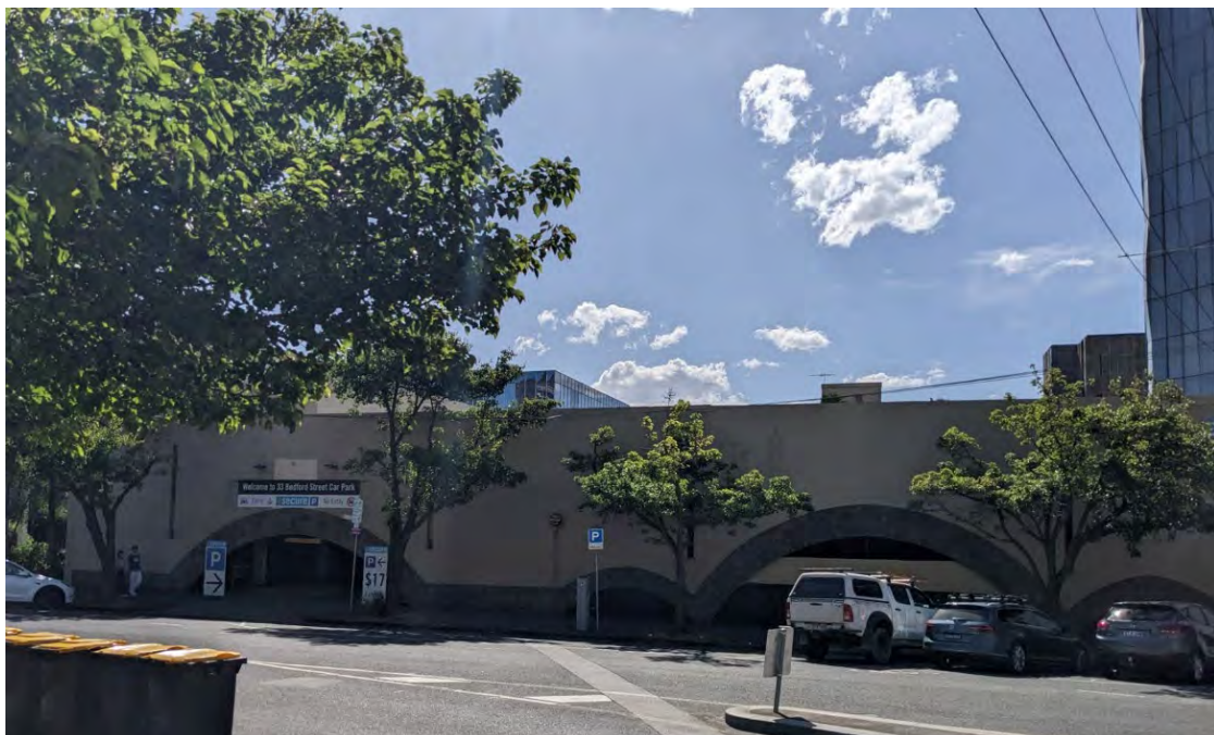
Figure 4: Subject site viewed from Bedford Street
