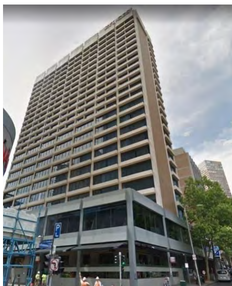
Figure 459. Former Bryson Centre, 174–192 Exhibition Street, Melbourne (HO1332 City of Melbourne). (Source: GML, 2020)
