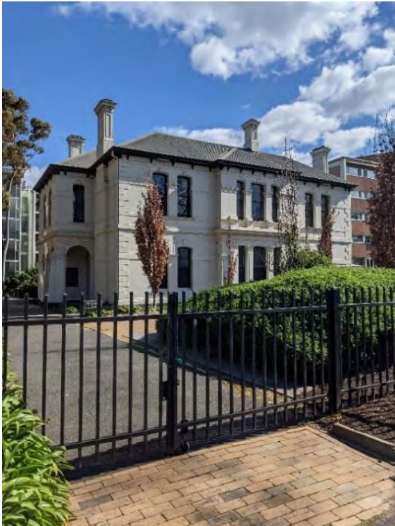
Figure 292. View of Greycourt from Royal Parade. (Source: GML, August 2022)
