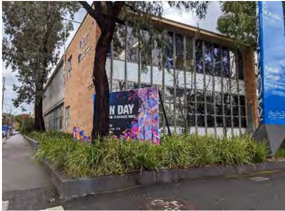
Figure 17. Primary (east) façade of the Sissons Building when viewed from the corner of Walker Street and Royal Parade. (Source: GML)
