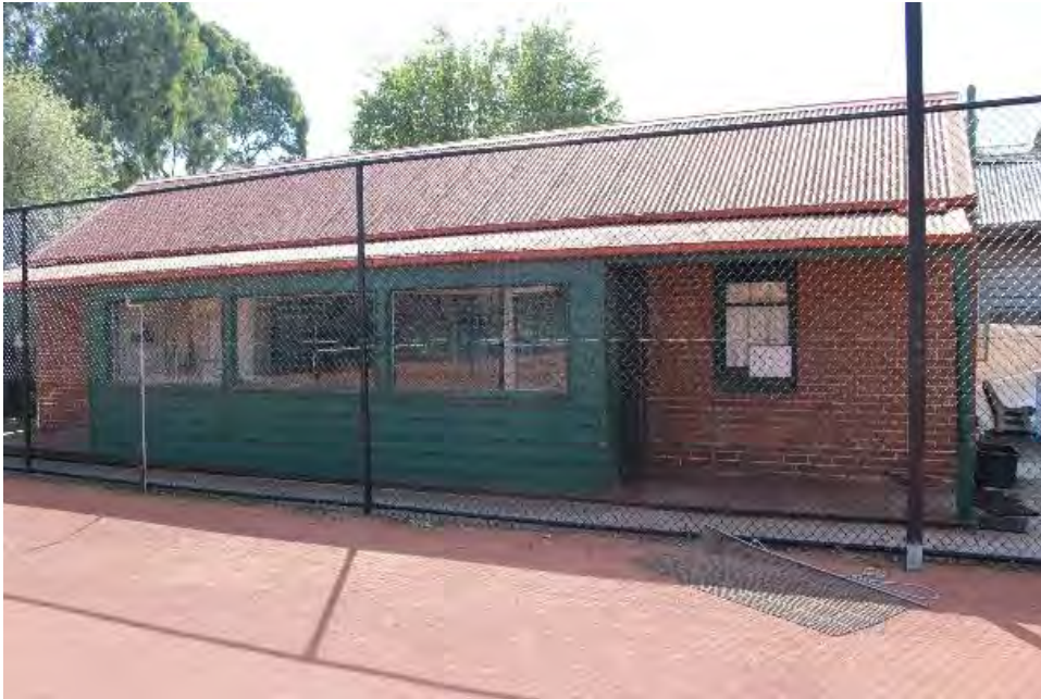
Figure 219. South elevation of the 1935 clubhouse. (Source: courtesy Parkville Tennis Club)
