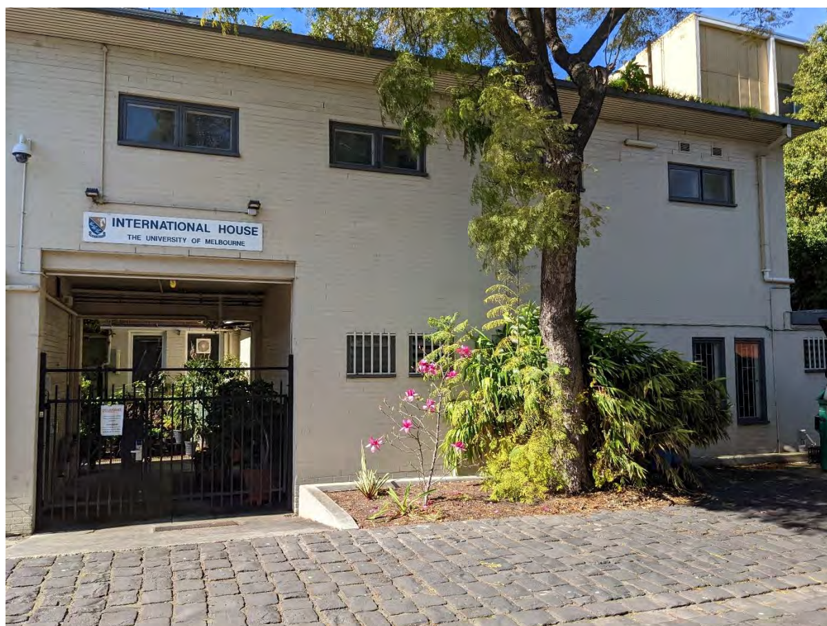
Figure 331. View of the West Wing from Mile Lane. (Source: GML, August 2022)
