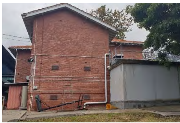
Figure 157. Director's Residence (east elevation). (Source: GML, December 2022)
