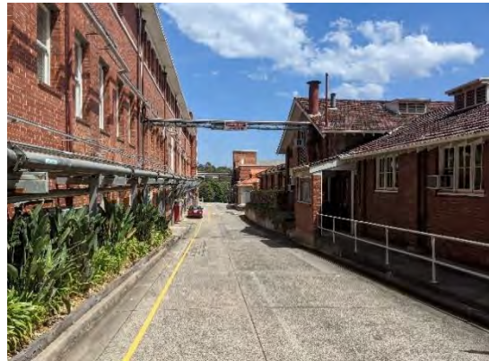
Figure 167. View of Block 5 (left) looking south, depicting the essential utility infrastructure connecting the Electrical Maintenance Building. (Source: GML, December 2022)
