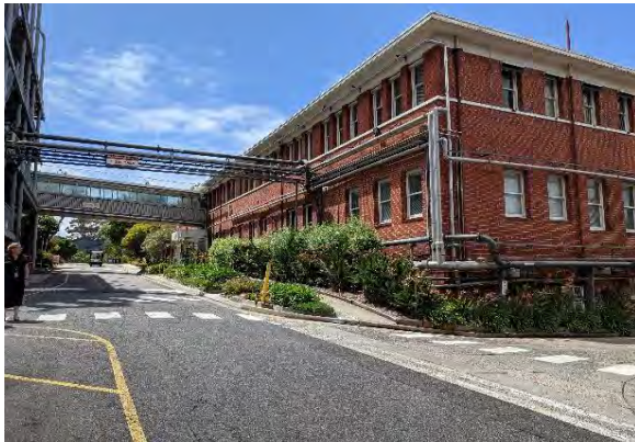
Figure 166. View of Block 5 looking east, with the elevated walkway connecting to South Block over Fourth Avenue in the background. (Source: GML, December 2022)
