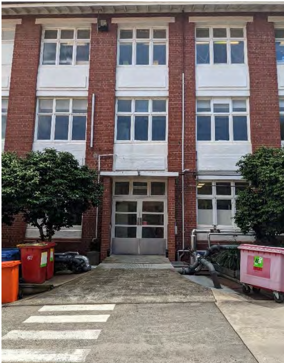
Figure 160. South Block (south elevation) depicting the main entrance from the south (primary) façade. (Source: GML, December 2022)
