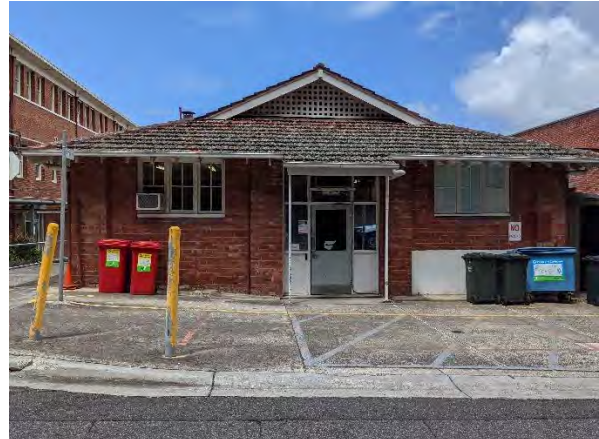
Figure 163. Electrical Maintenance Workshop (north elevation). (Source: GML, December 2022)
