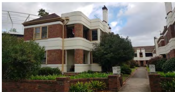
Figure 358. View towards the southern wing of the main building. (Source: GML Heritage, 2022)
