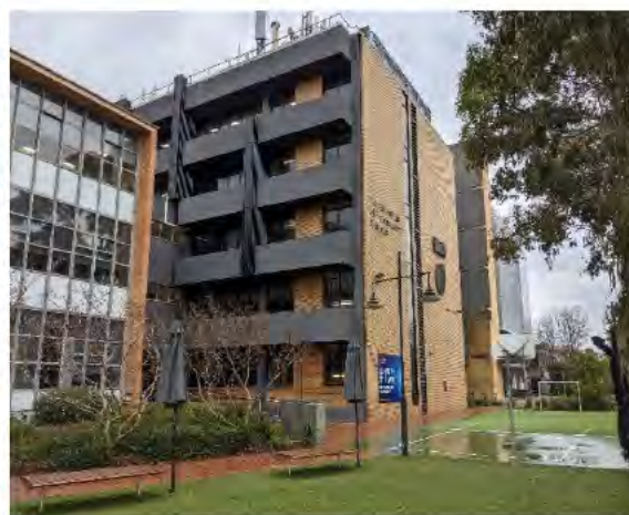
Figure 33. South elevation of the Manning Building. (Source: GML)
