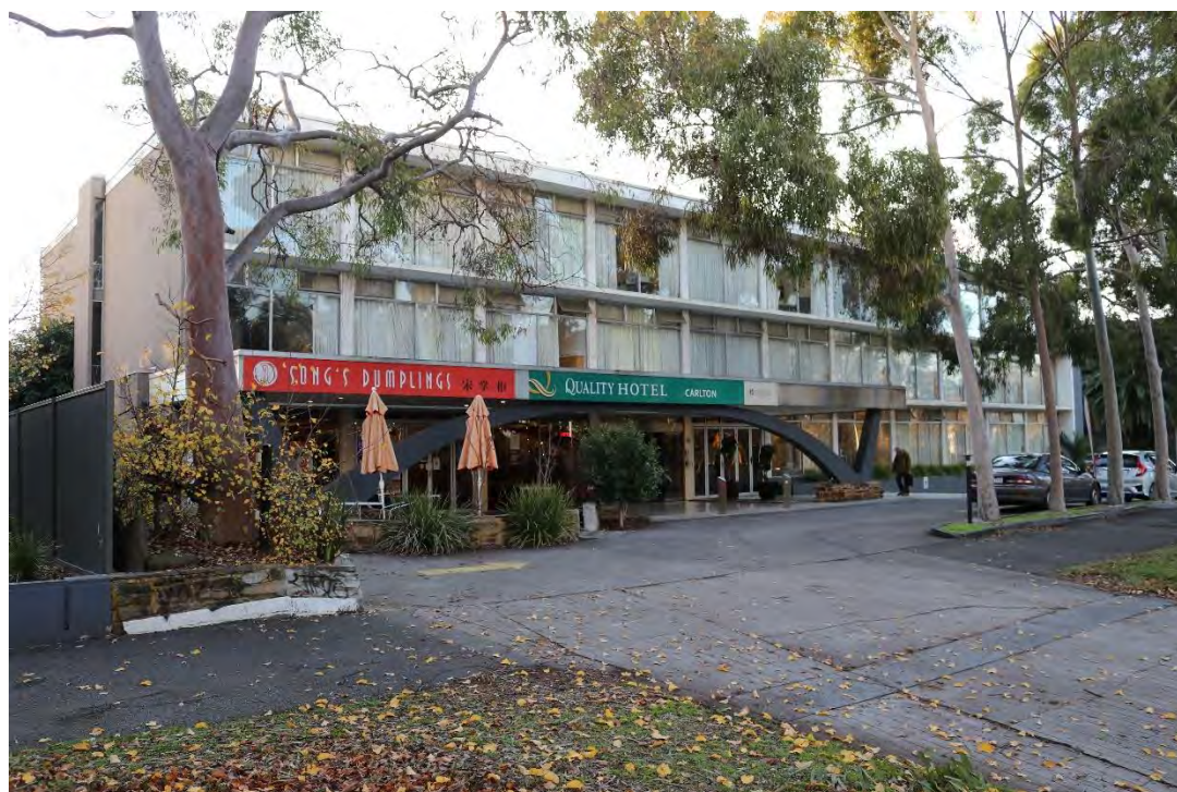
Figure 453. The principal façade at the former Motel Parkroyal. (Source: GML, 2022)
