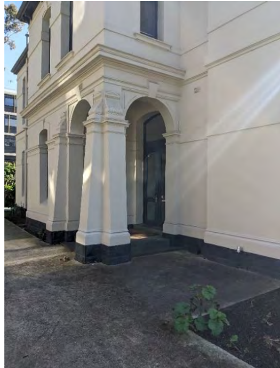
Figure 293. View of southern side porch with buttresses. (Source: GML, August 2022)
