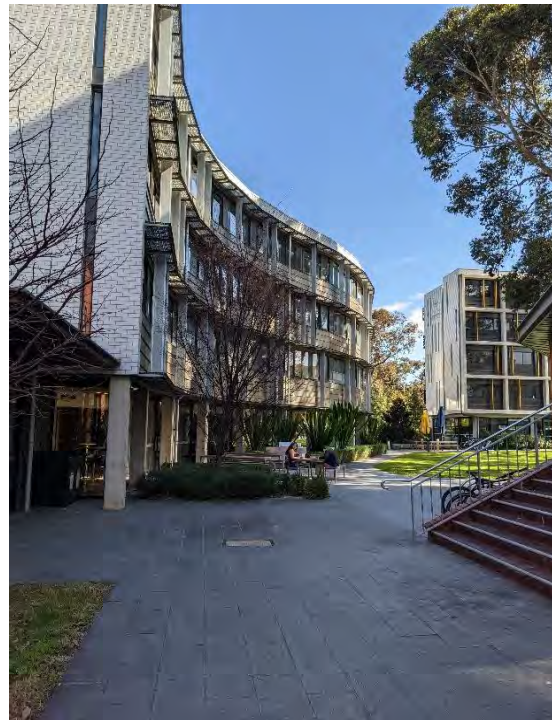
Figure 338. View of the George Hicks Building looking west. (Source: GML, August 2022)
