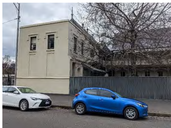
Figure 300. View of the 1937 addition, with partial view of the 1907 addition behind. (Source: GML, August 2022)
