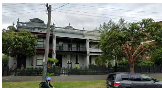
Figure 251. 272–278 The Avenue, Parkville. (Source: GML, 2022)
