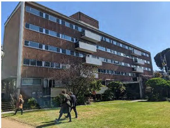
Figure 320. Eastern view of Samuel Wadham Wing. (Source: GML, August 2022)
