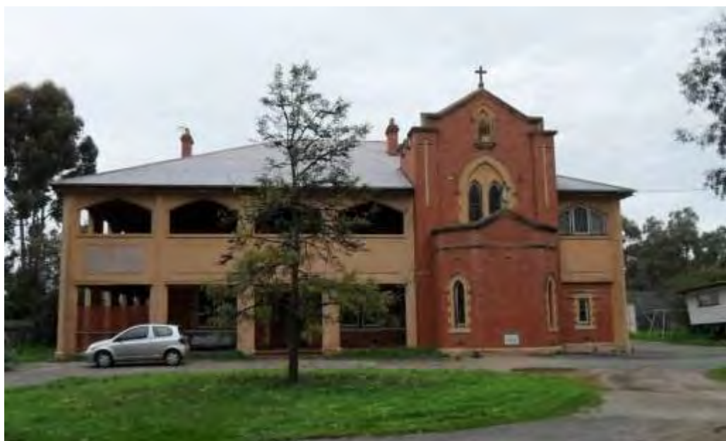
Figure 207. Former Catholic convent at 7 Lyle Street, Warracknabeal, constructed 1929–30. (Source: Yarriambiack Shire Council)
