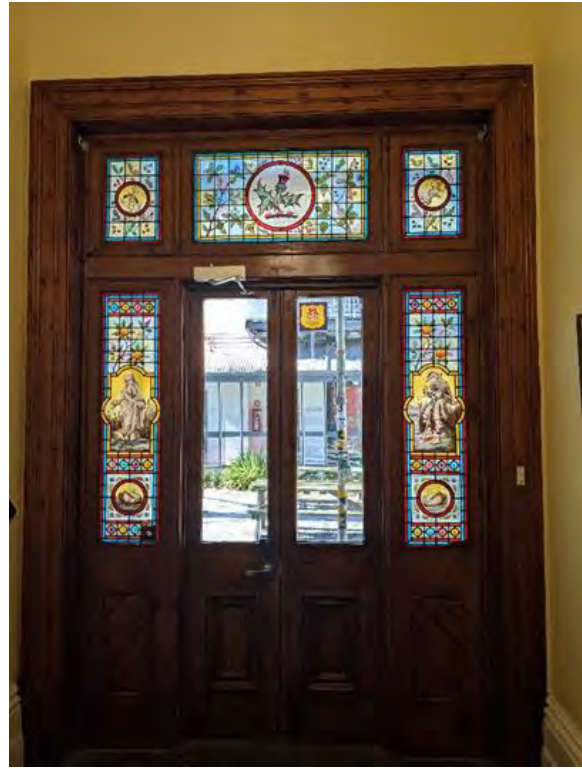
Figure 303. Internal view of the front door of the original 1886–87 house. (Source: GML, August 2022)
