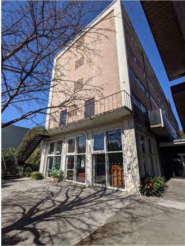
Figure 324. North side of the Samuel Wadham Wing showing the Junior Common Room area. (Source: GML, August 2022)
