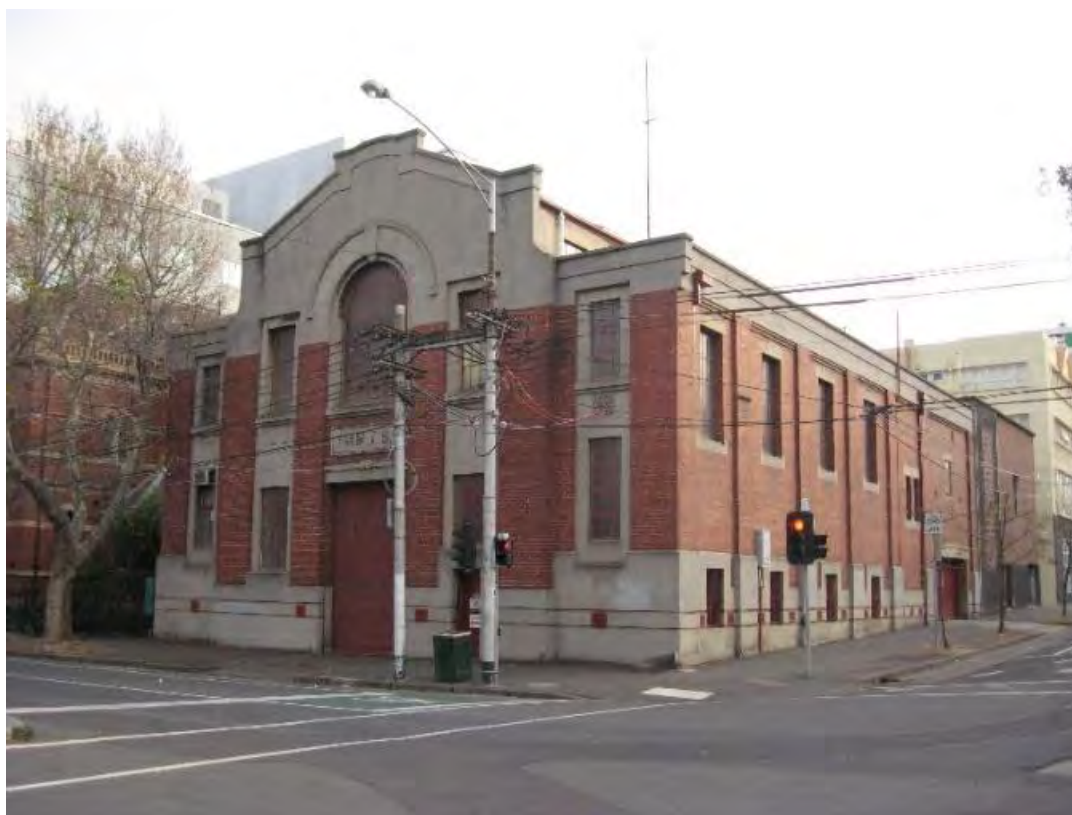
Figure 180. Carlton Tram Substation, Carlton. (Source: City of Melbourne)
