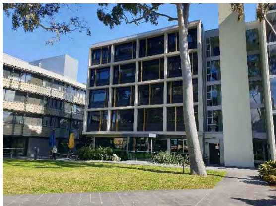
Figure 336. Partial view of the Founders Building, with the George Hicks Building to the left. (Source: GML, August 2022)
