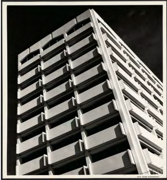
Figure 375. Exterior view of the new Zebra Motel, Parkville (c1970–75), looking straight up at floors of the motel. Photograph by John Squire. (Source: State Library Victoria, Accession No. H2016.34/104)
