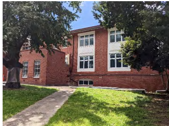
Figure 152. East Block west elevation, showing additions to the southwest area of the building. (Source: GML, December 2022)
