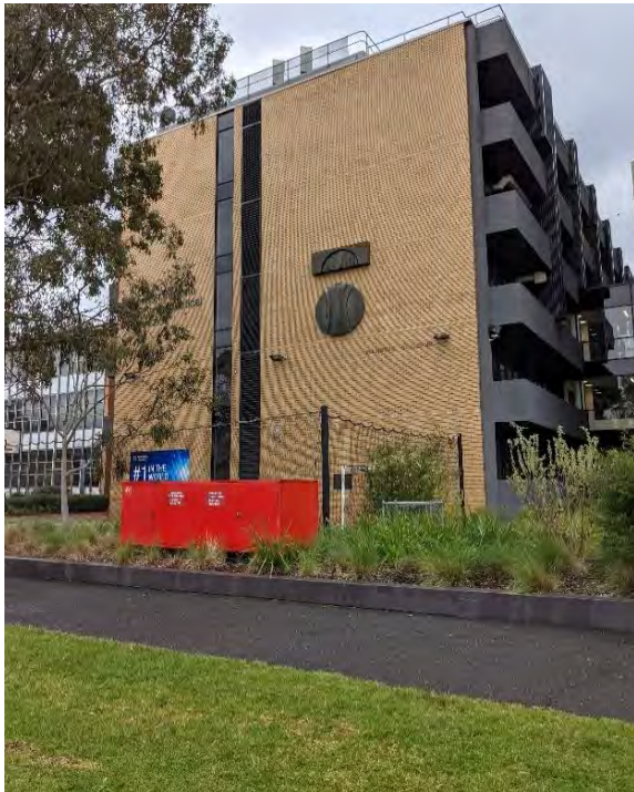
Figure 34. View of the primary (east) elevation of the Manning Building from Royal Parade. (Source: GML)
