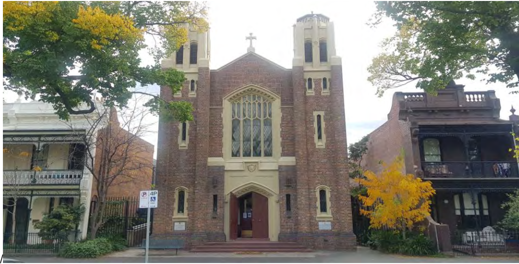
Figure 196. View showing St Carthage's Church in its immediate setting, seen from Royal Parade. (Source: GML Heritage)
