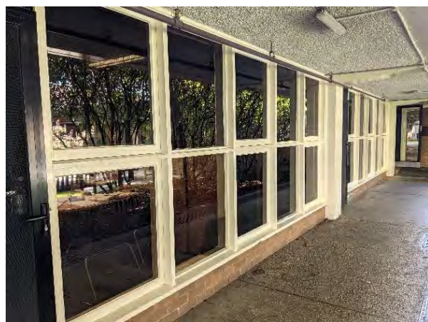
Figure 316. View of the lower level (east side) with main entrance door in the background. (Source: GML, August 2022)
