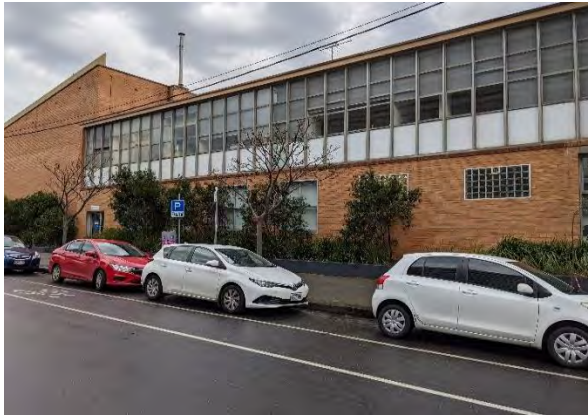
Figure 28. Sissons Building (south elevation) when viewed from Walker Street. (Source: GML)
