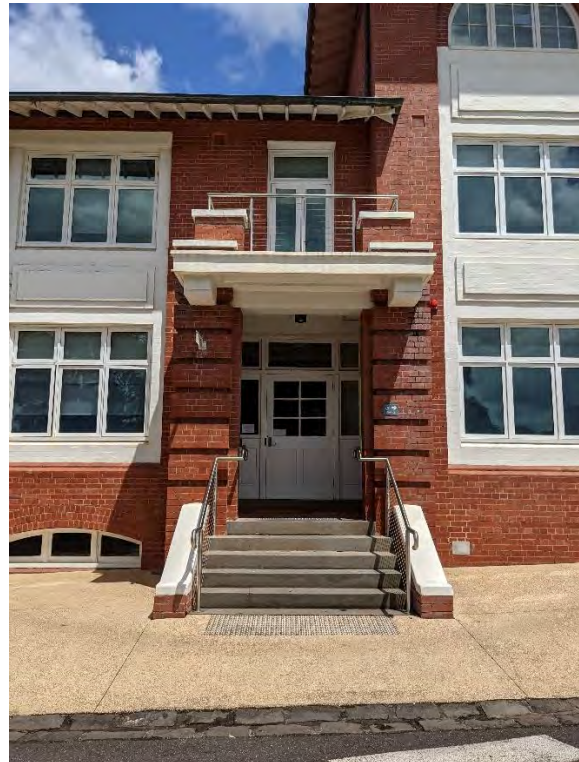
Figure 150. East Block (east elevation) showing the main entrance. (Source: GML, December 2022)
