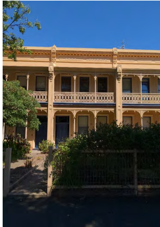
Figure 247. View of Park Terrace from Royal Parade. (Source: GML, 2022)
