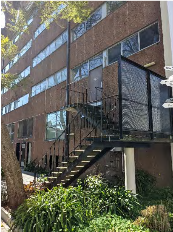
Figure 322. Samuel Wadham Wing (west side). Windows throughout the building are typically sliding windows in aluminium frames. (Source: GML, August 2022)
