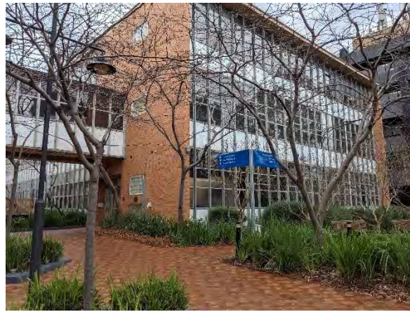
Figure 20. Primary (east) façade of the Scott Building when viewed from Royal Parade. (Source: GML)
