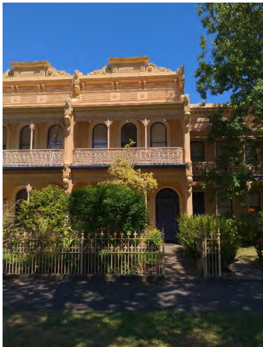
Figure 236. View of 165 Royal Parade, and a partial view of the neighbouring Park Terrace, which is set back behind the building line. (Source: GML, 2022)
