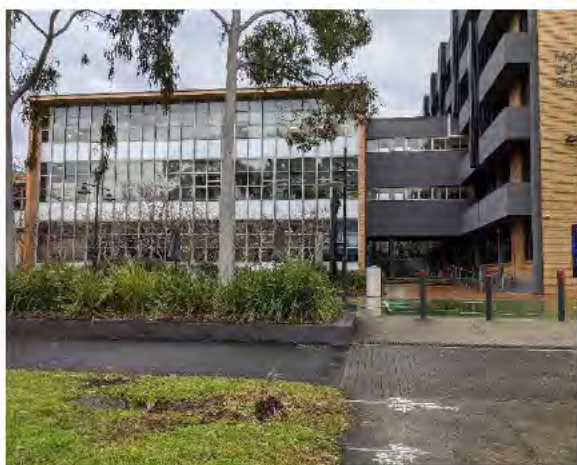
Figure 32. View of Scott and Manning buildings from Royal Parade. (Source: GML)
