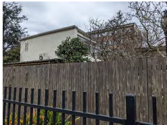
Figure 319. Partial view of the Warden's Residence from Royal Parade. (Source: GML, August 2022)
