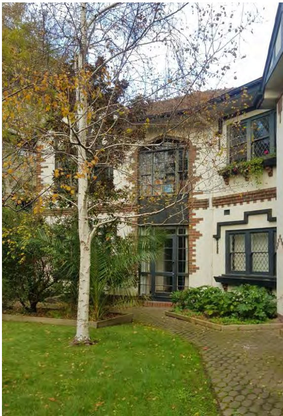
Figure 420. Detail showing the rear wing facing towards the integrated courtyard garden. (Source: GML Heritage, 2022)
