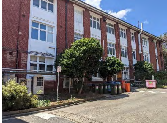
Figure 159. South Block (south elevation) viewed from Fourth Avenue. (Source: GML, December 2022)
