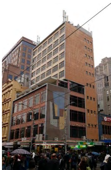
Figure 458. Former Hosie's Hotel, 1–5 Elizabeth Street, Melbourne (HO1327 City of Melbourne). (Source: GML, 2020)
