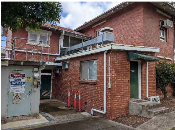
Figure 156. Director's Residence (east elevation). (Source: GML, December 2022)
