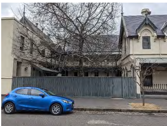
Figure 299. View of the internal courtyard and U-shaped plan of the building additions from Leonard Street. The 1904–05 addition is located at the centre, with the 1907 and 1937 additions situated to the east. (Source: GML, August 2022)
