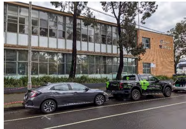
Figure 27. Sissons Building (south elevation) when viewed from Walker Street. (Source: GML)
