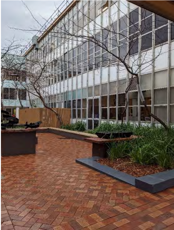
Figure 22. Scott Building (south elevation) when viewed from the internal courtyard. (Source: GML)
