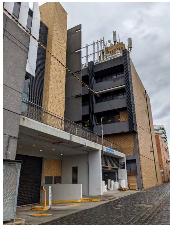
Figure 37. Manning Building (north elevation) when viewed from Mile Lane. (Source: GML)
