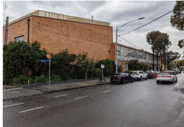
Figure 29. Sissons Building (south elevation) when viewed from Walker Street. (Source: GML)
