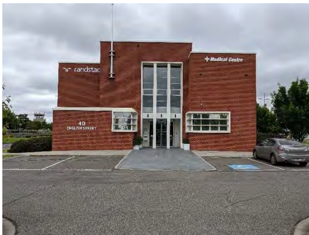
Figure 184. Former Area Approach Control Centre (Building 79), Essendon Airport. (Source: GML, 2022)
