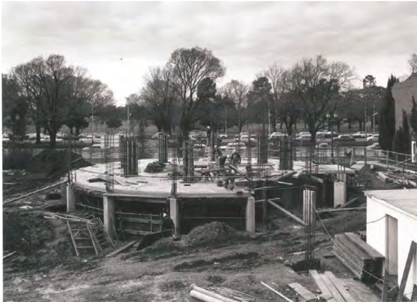
Figure 285. Scheeps Wing under construction, August 1971. (Source: International House Archives)
