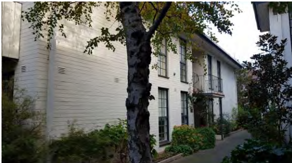
Figure 424. View showing the northern elevation of the later residential addition facing the central path. (Source: GML Heritage, 2022)
