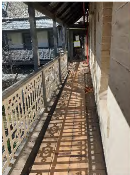
Figure 307. View from the verandah looking east along the 1904–05 addition, with a partial view of the 1907 addition (left). (Source: GML, August 2022)
