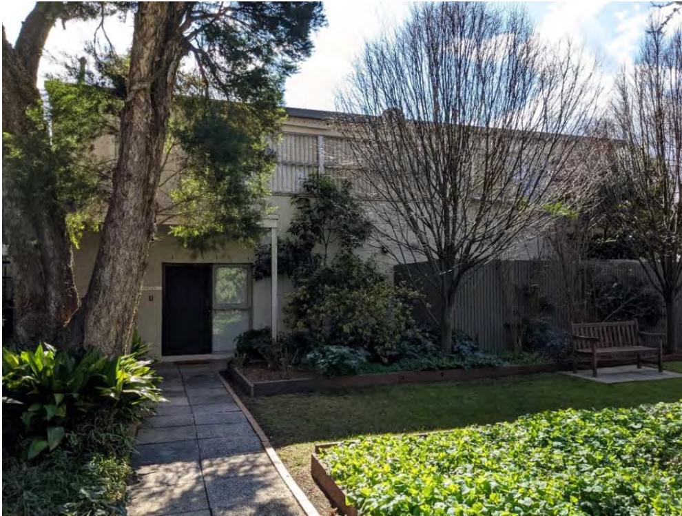
Figure 317. South elevation of the Warden's Residence viewed from in front of the Samuel Wadham Wing. (Source: GML, August 2022)
