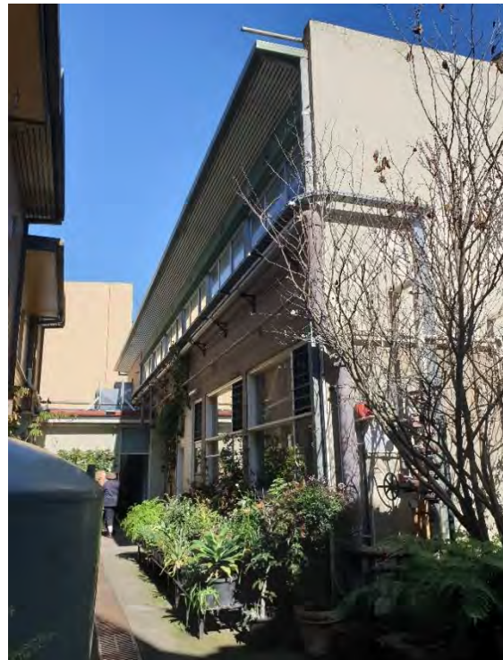
Figure 330. View of the West Wing. (Source: GML, August 2022)
