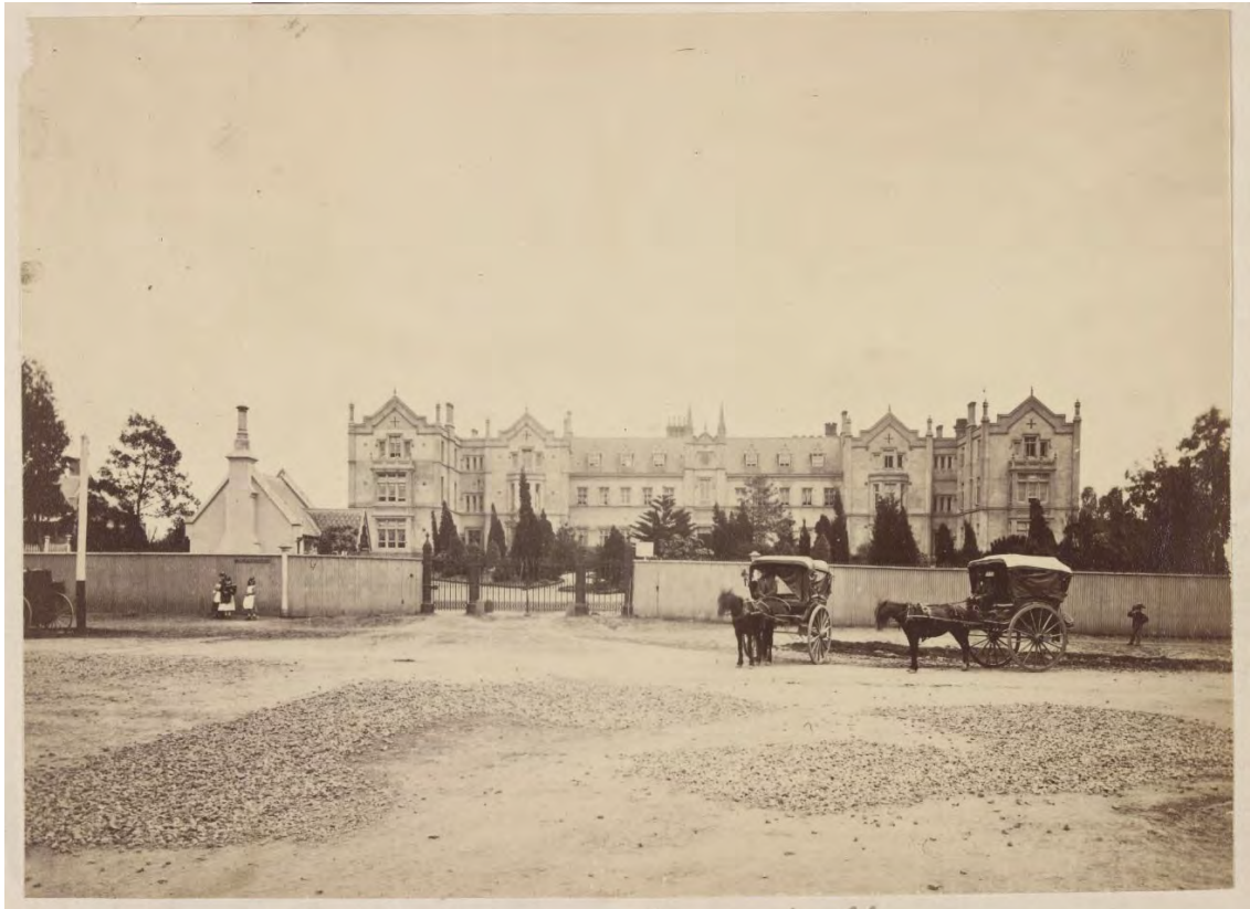
Figure 49 View of Benevolent Asylum, c. 1870, at intersection of Victoria and Curzon streets Source: D McDonald, photographer, H4249, State Library of Victoria
