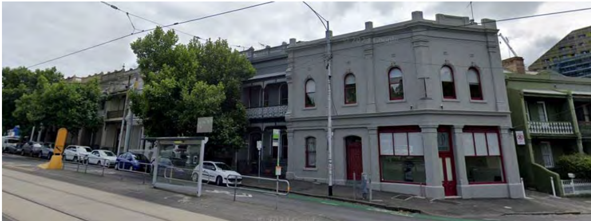
Figure 3 480-482 Abbotsford Street, North Melbourne (corner property)
