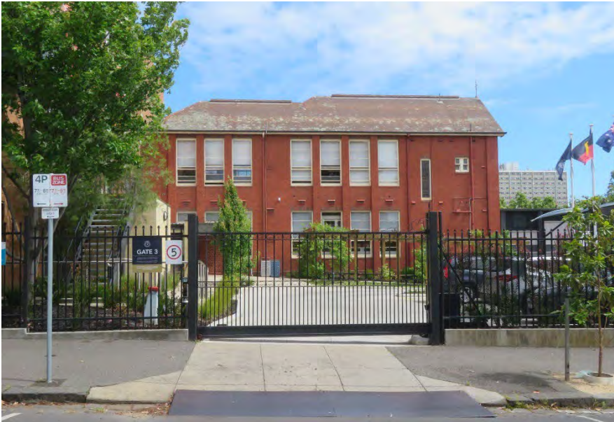
Figure 5 North elevation of 1940 School Building (facing Curran Street)
