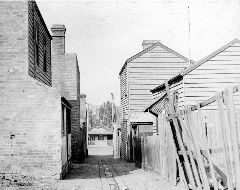
Figure 17 View south along Avon Place, 1935, with four timber residences fronting this street. A house on Haines Street can be seen at the end of the lane Source: H2001.291/54, F Oswald Barnett collection, State Library of Victoria
