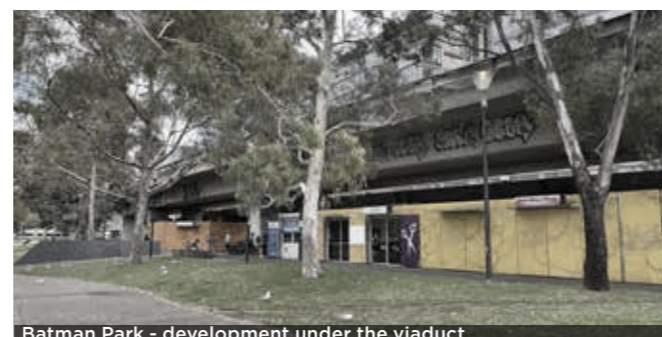
Batman Park - development under the viaduct
