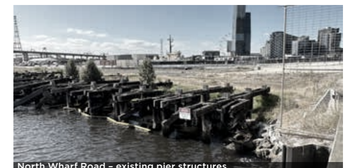
North Wharf Road - existing pier structures
