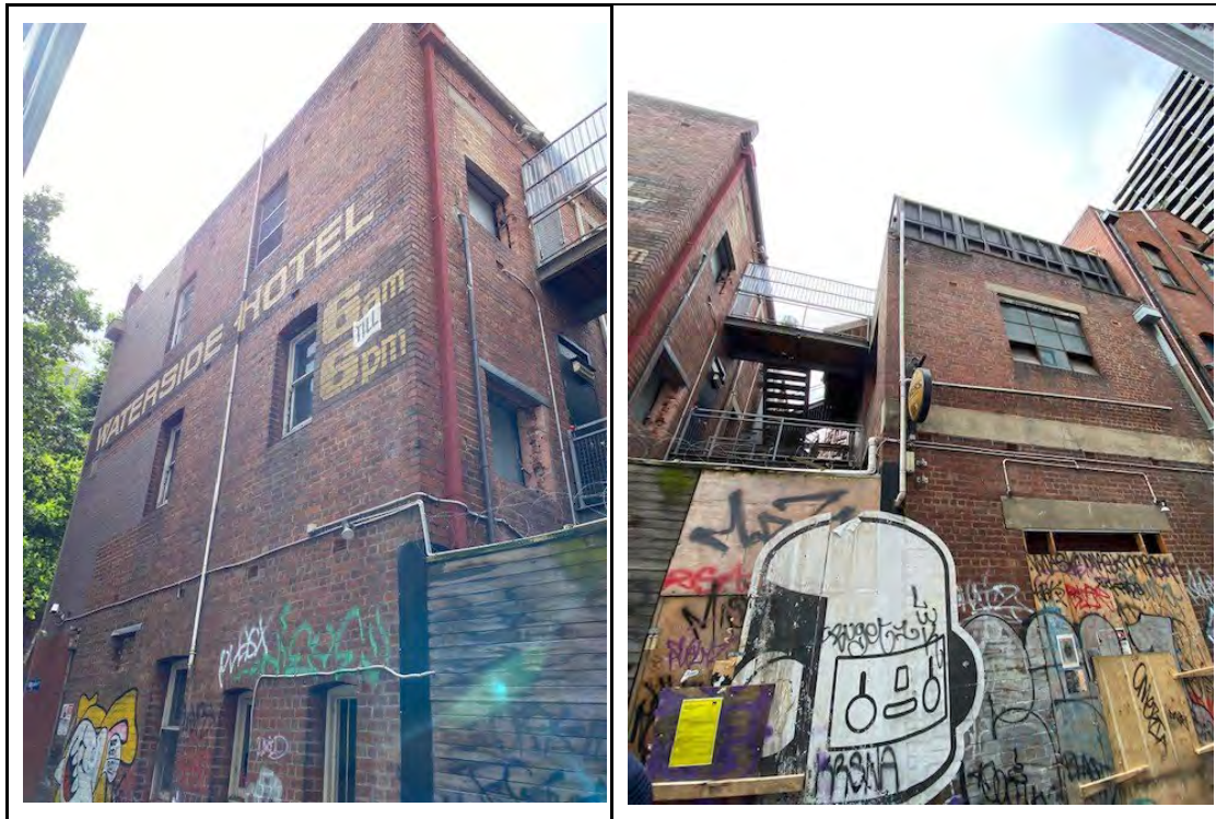
Figure 5: Mercantile Place Frontage
