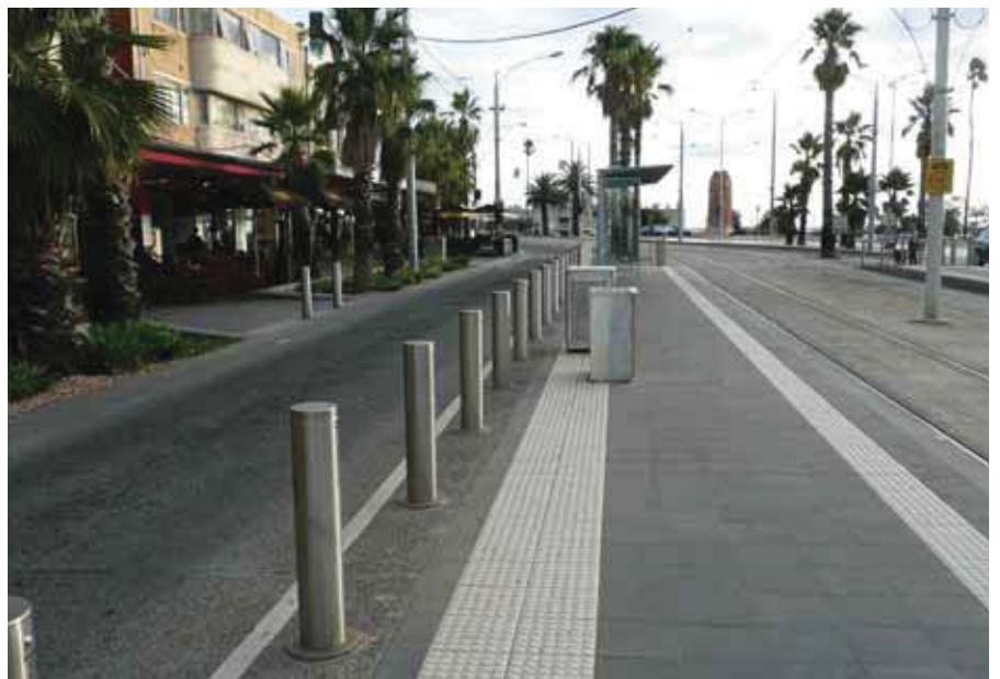
Fig 7.2 Level access tram stop showing permeable access to footpath in StKilda
