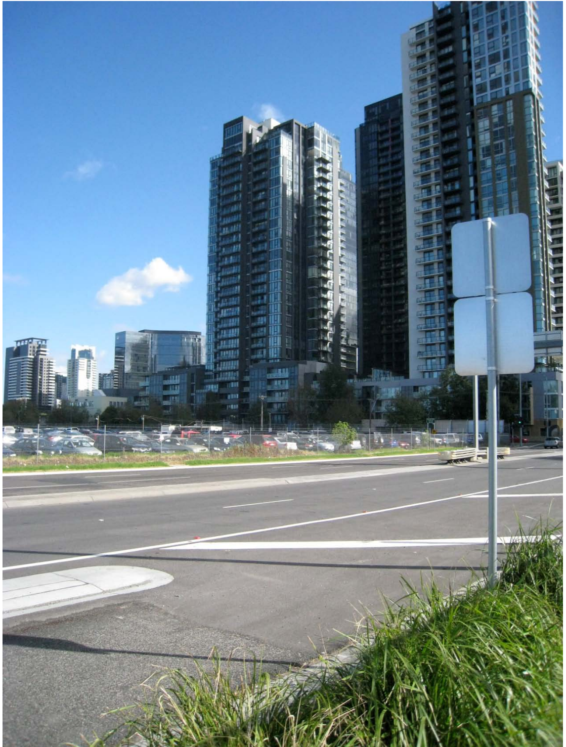
Figure 4. Despite being in the centre of Melbourne, these buildings overlook only an enormous carpark.
