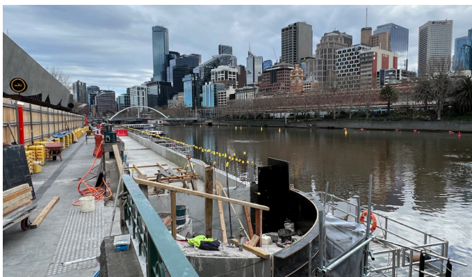
Stage one Southbank Promenade upgrade works
