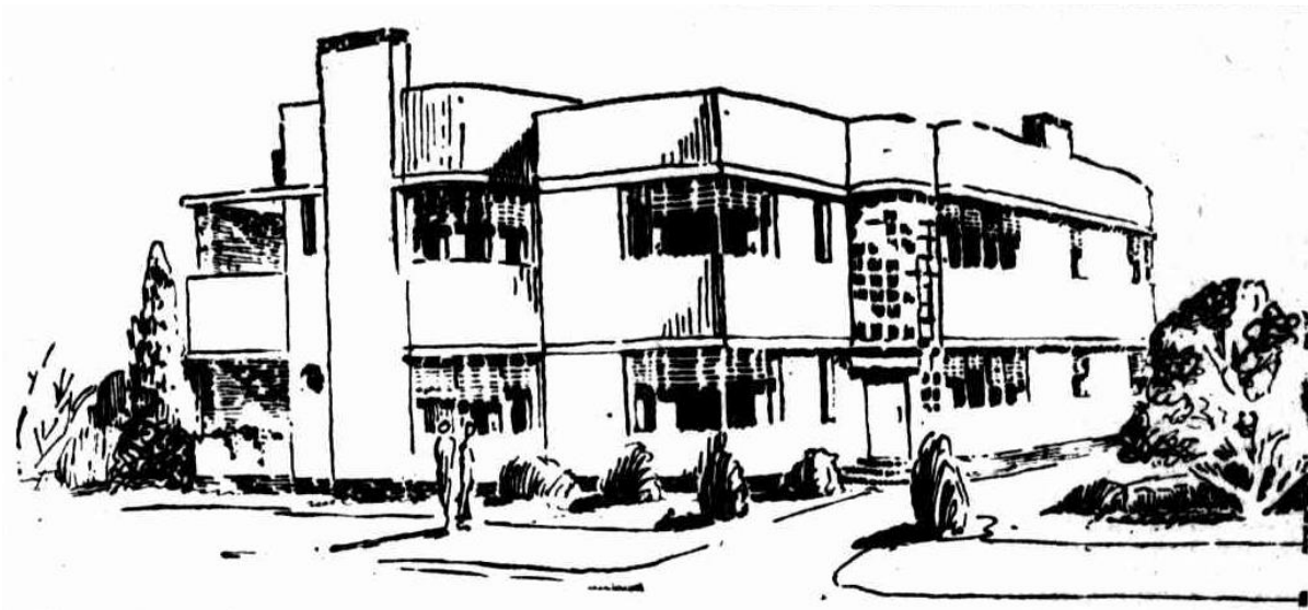
Figure 3.38 Moderne block of flats in Clowes Street, built in 1937, built using a method of cantilevered construction and with extensive use of glass. (Source: Age , 9 February 1937, p. 17)
