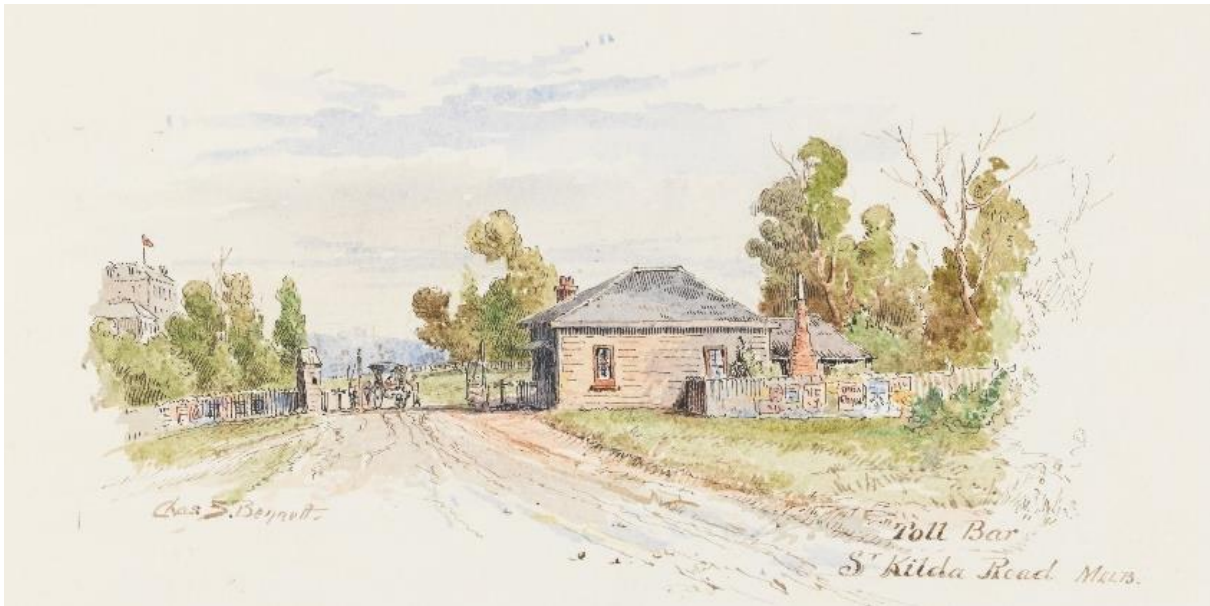
Figure 3.58 Toll booth, St Kilda Road, looking towards town, painted by Charles Bennett, [n.d.], c.1880s. (Source: State Library of New South Wales)
