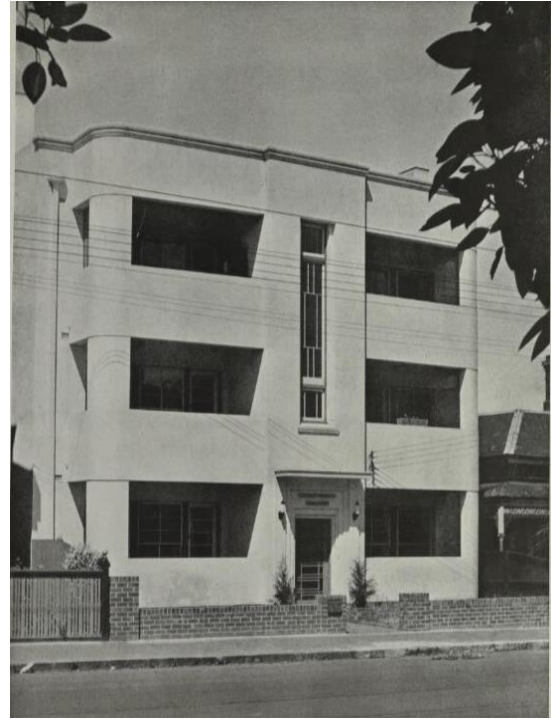
Figure 3.45 Block of flats in Domain Road designed by Marcus Martin. (Source: The Home: An Australian quarterly , vol. 17, no. 4, 1 April 1936)
