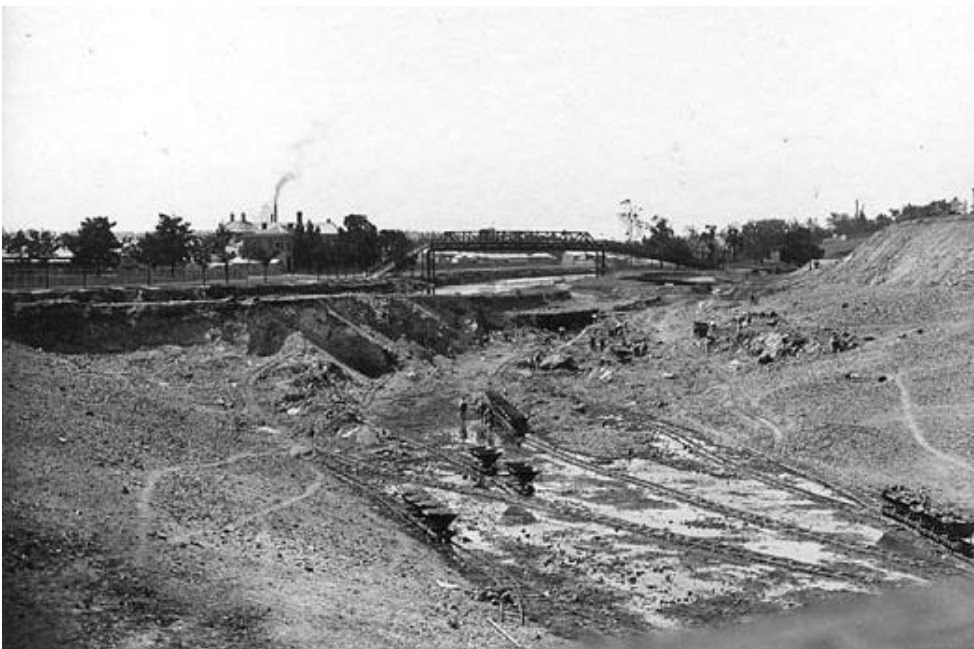
Figure 3.12 Work on the realignment of the Yarra River 1898. (Source: University of Melbourne Archives; copyright restrictions may apply)
