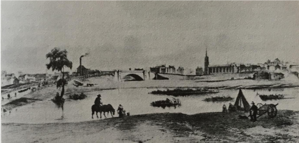
Figure 3.21. View from the south bank of the Yarra, showing temporary tent accommodation, early 1850s. (Source: Shirley Roberts, Charles Hotham , p. 97)
