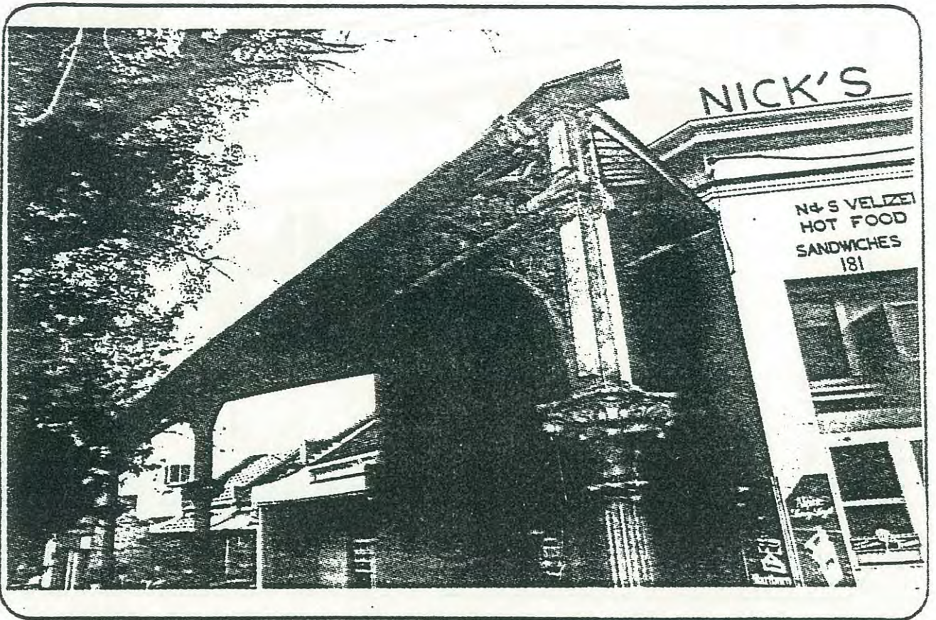
Corporation Iron Street Verandah, 181 Adderley Street, 1889 (incomplete)
