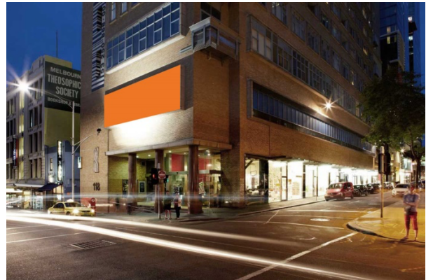
Image courtesy of Hero Apartment Building.
