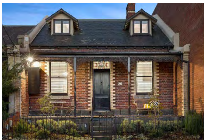
20 Wimble Street, Parkville - before and after paint removal
