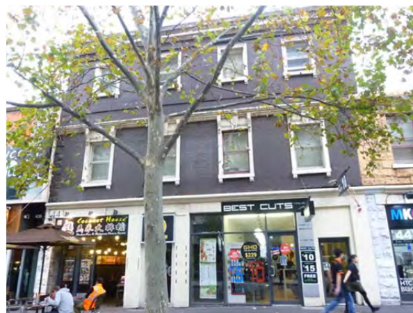
Former Royal Saxon Hotel, nos 441-445
