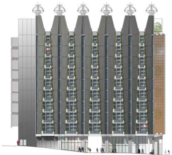
Figure 7: Rendering of north façade showing six wind-assisted extraction turbines.
