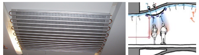
Figure 8. Chilled ceiling panel providing radiant cooling
