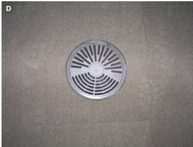
D: Floor mounted swirl diffuser, with rotating occupant controlled grill for directing and varying air flow.
