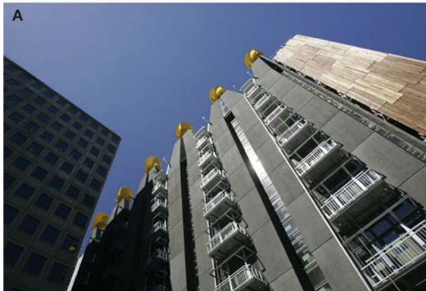
A: Finished north façade prior to placement of the plants on balconies to create a living façade. Darkened north exhaust flue chimneys leading to the roof mounted air extraction and electricity generating wind turbines are also shown.
