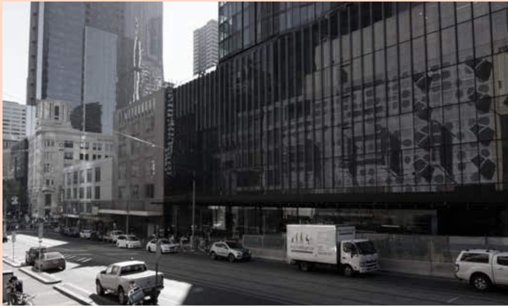
Figure 24 This continuous reflective glass frontage extends over 60m in length or one third of a block in the Hoddle Grid. The flatness and length of the facade erodes the characteristic grain, rhythm and visual interest of the streetscape.
