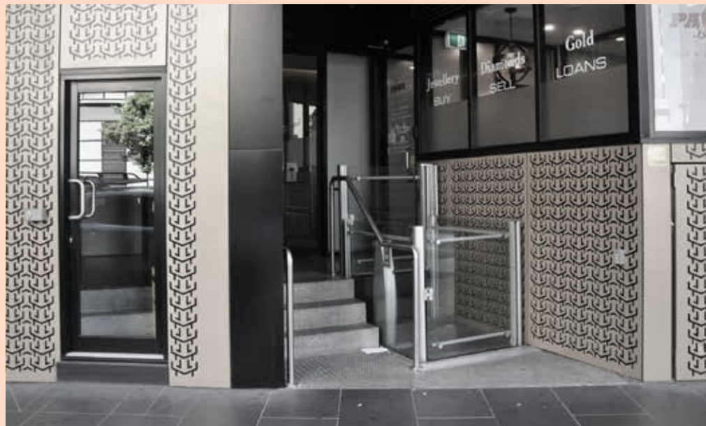
Figure 47 Platform lifts should be avoided within the public realm, where they gather litter and result in unsafe spaces.
