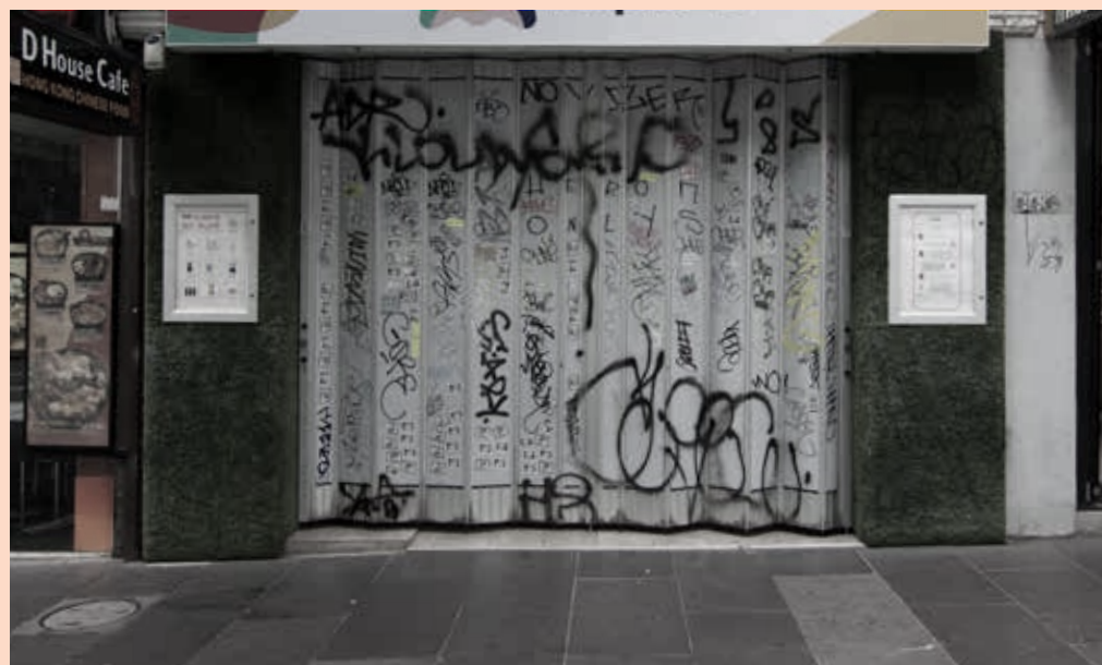
Figure 48 Solid metal shutters present poorly to the public realm when closed and are prone to graffiti and damage.
