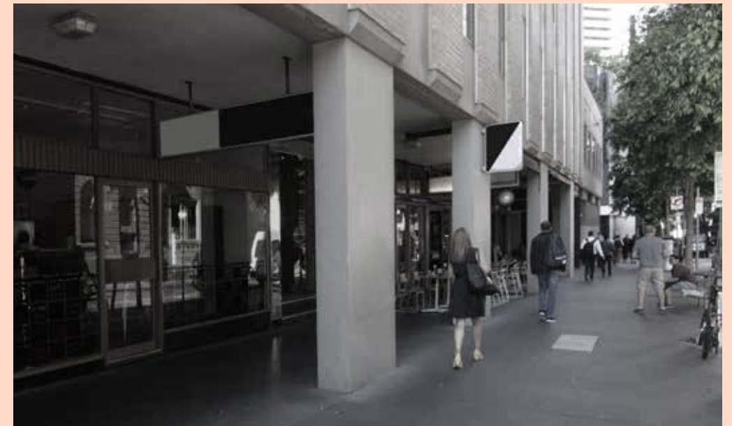
Figure 20 Low height colonnades with broad columns at the street edge can limit views through to the building interior and negatively impact upon the attractiveness and success of retail spaces.
