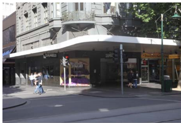
Figure 405 altered ground level
