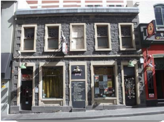
Figure 281 68-70 Little Collins Street
