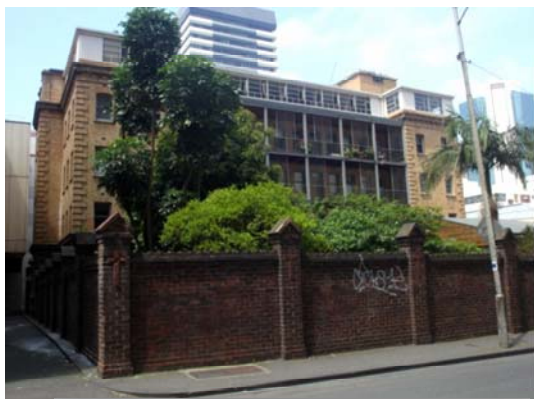
Figure 314 326 Lonsdale Street (part)-north elevation with added steel framed verandah and roof addition.
