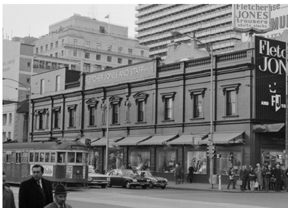
Figure 202 Flinders Street elevation 1960s (State Library of Victoria collection H36133)
