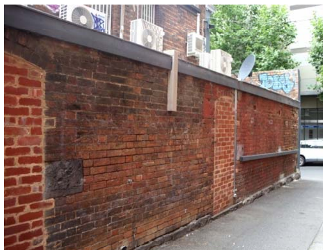
Figure 360 brick wall on lane, openings changed
