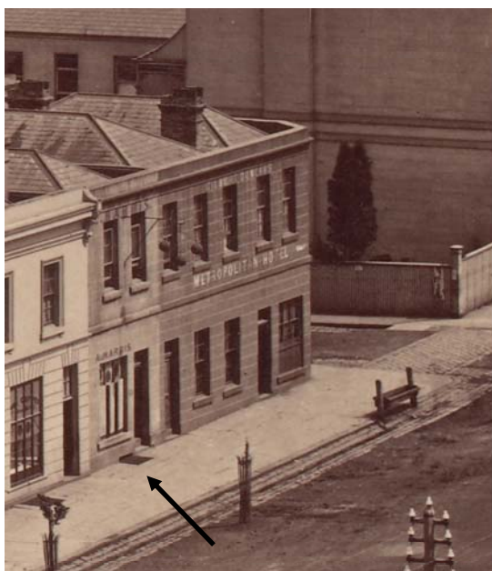
Figure 457 View of 261 William Street in the 1881 panorama, adjoining former Metropolitan Hotel building.
