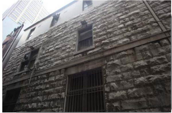
Figure 195 360-372 Flinders Street, stone west elevation onto lane.
