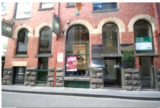
Figure 239 106-112 Hardware Street, ground level
