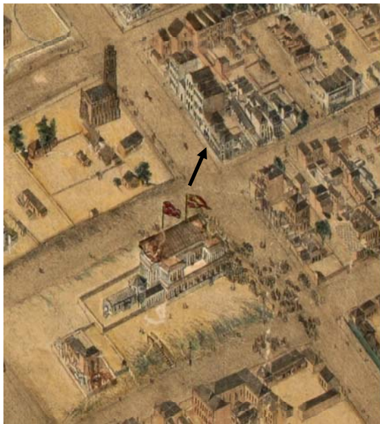
Figure 461 DeGruchy & Leigh 1866: isometric detail with hotel row and 'Crystal palace' exhibition building.
