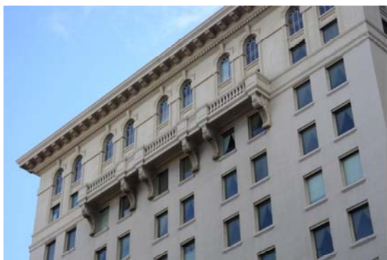
Figure 392 122-132 Spencer Street, detail upper level
