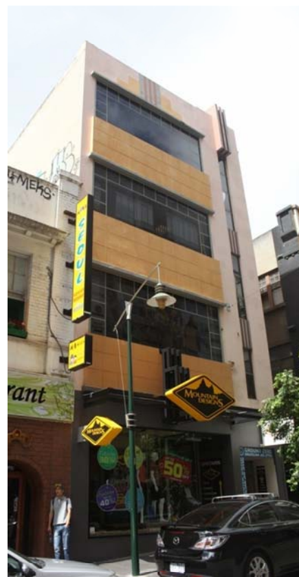
Figure 273 373-375 Little Bourke Street
