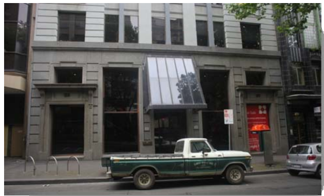
Figure 336 20-26 Queen Street, ground level
