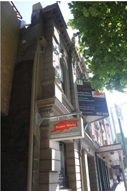
Figure 214 520-522 Flinders Street, showing stone west wall behind cemented façade
