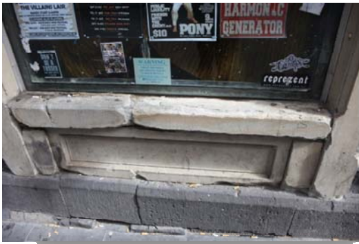
Figure 282 68-70 Little Collins Street- valuable stonework
