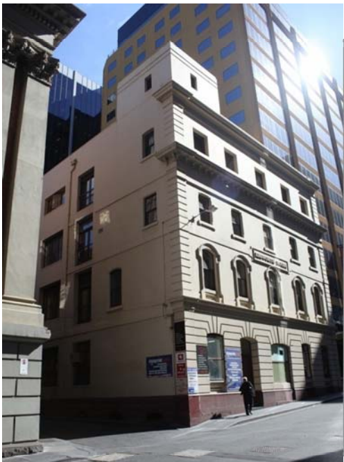
Figure 289 538-542 Little Collins Street
