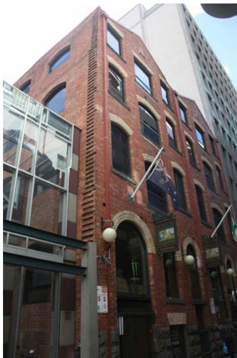
Figure 238 106-112 Hardware Street, with atrium on north
