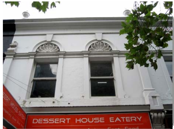
Figure 415 309-325 Swanston Street, upper level detail, shell motifs and inverted consoles.
