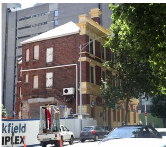
Figure 437 427-433 Swanston Street, rear
