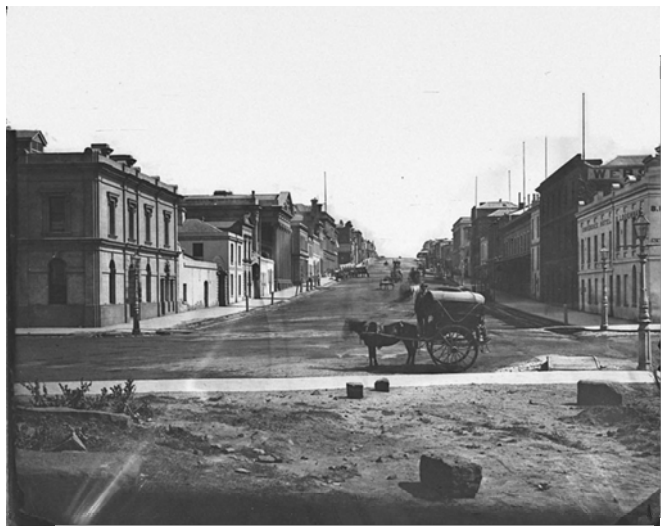
Figure 201 View north up Queen Street c1870-1875 showing original east facade (Mitchell Library Holterman Collection)
