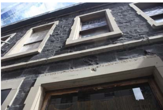
Figure 283 68-70 Little Collins Street
