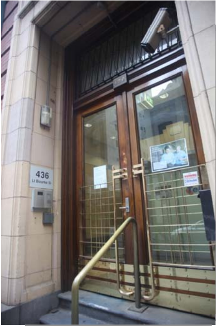
Figure 278 Entrance, high integrity to construction.
