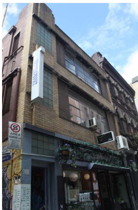
Figure 260 361-363 Little Bourke Street
