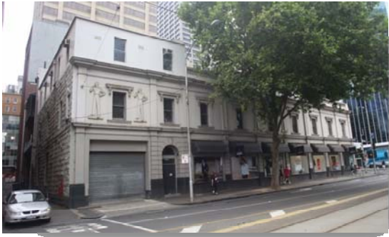
Figure 192 360-372 Flinders Street, showing added floor
