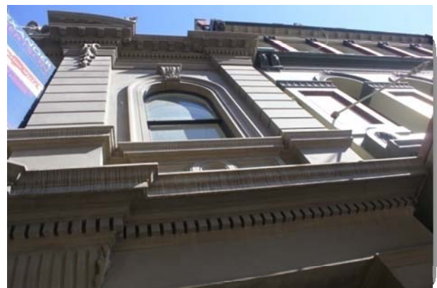
Figure 216 520-522 Flinders Street, deeply modelled upper level adjoining former coffee palace.
