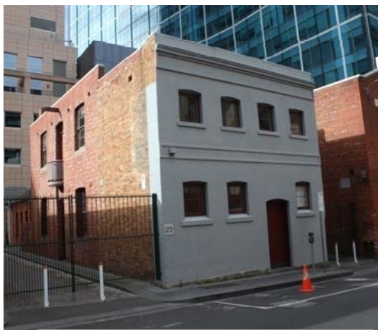
Figure 294 25 Little Lonsdale Street, with 20 th century wing at rear.
