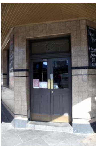
Figure 206 508-510 Flinders Street, corner entry with tiled facade and leadlight glazing.
