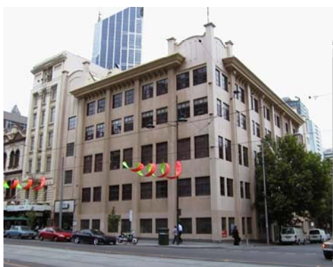
Figure 431 411-423 Swanston Street, 1990s, (MCC)
