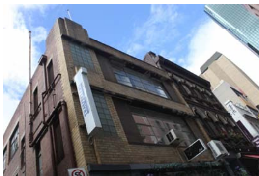
Figure 261 361-363 Little Bourke Street, upper level
