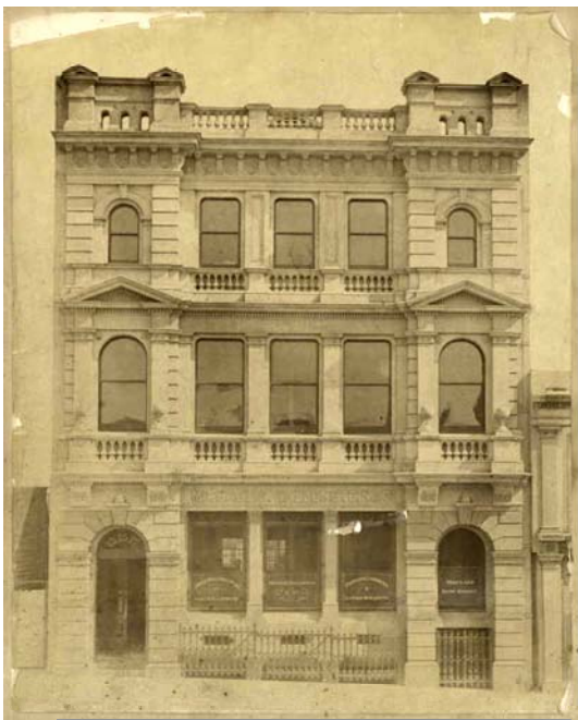
Figure 327 Former Michaelis Hallenstein building on site (Picture Victoria)
