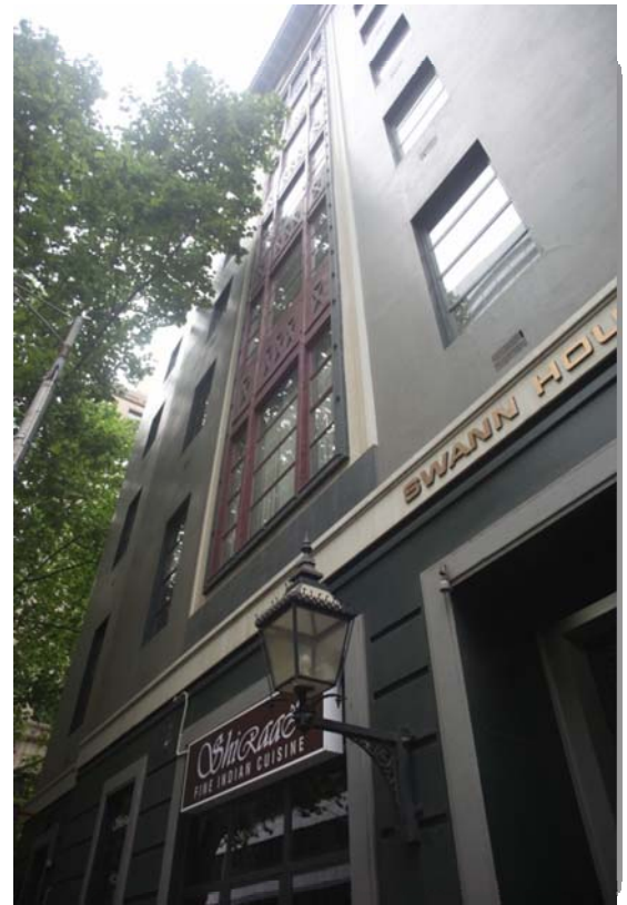
Figure 442 22-32 William Street, central facade motif
