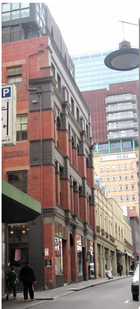
• Figure 6 Edwardian-era adjoining building
