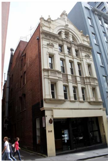
Figure 264 362-364 Little Bourke Street
