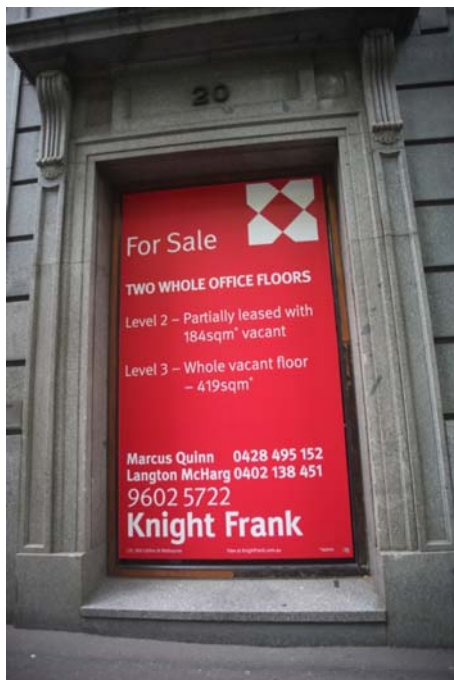
Figure 335 20-26 Queen Street, ground level detail.
