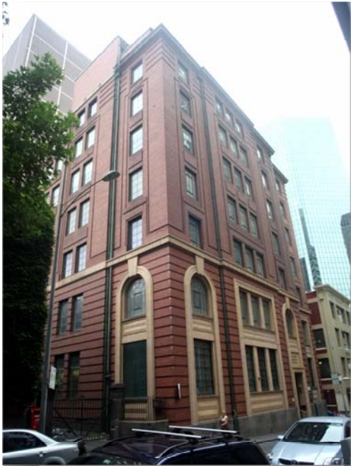
Figure 276 434-436 Little Bourke Street
