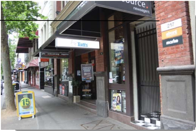
Figure 364 217-219 Queen Street, ground level, with stone pedestals to piers
