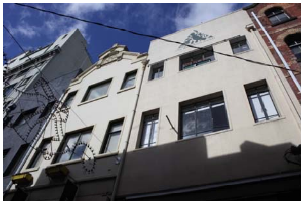
Figure 236 altered Hardware Street warehouses backing onto 4-6 Goldie Place, part of group.
