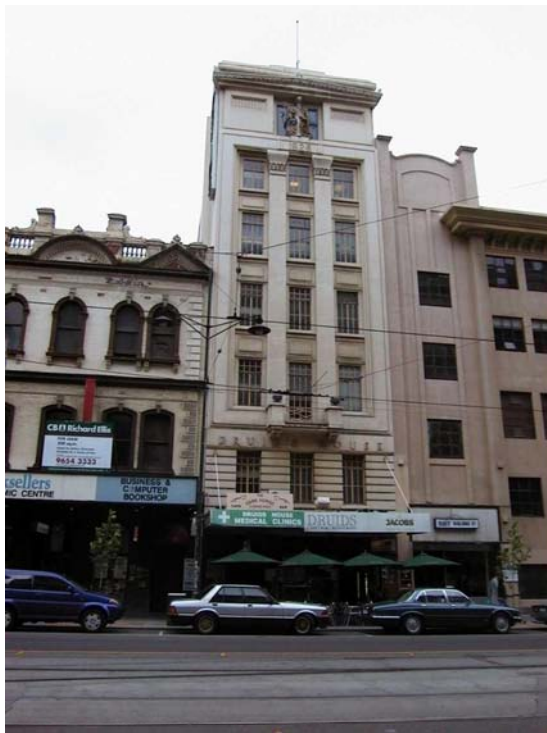
Figure 424 407-409 Swanston Street 1990s (MCC)
