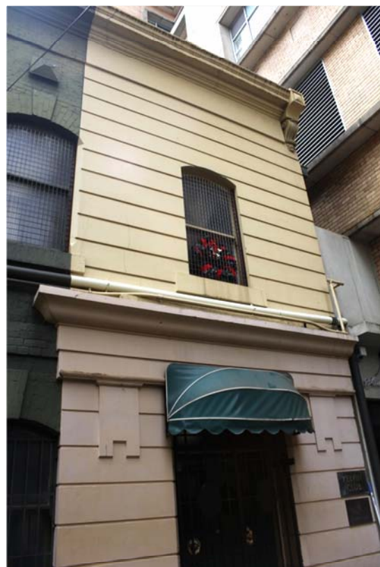
Figure 330 14-30 Melbourne Place: former radio station, now club entry, c1927.
