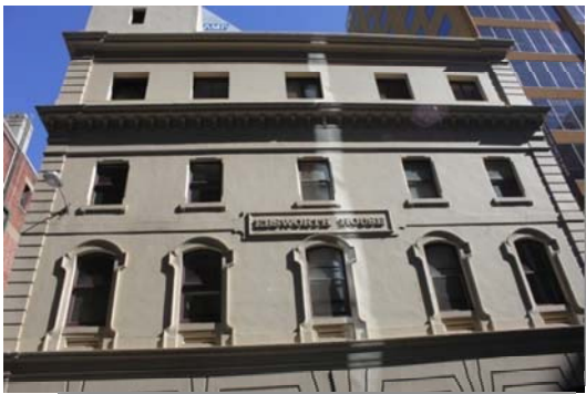
Figure 290 538-542 Little Collins Street upper level
