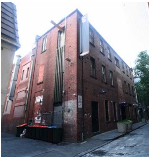
Figure 242 rear on Highland Lane with adjoining warehouse
