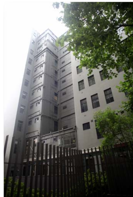
Figure 443 22-32 William Street, rear elevation, showing addition
