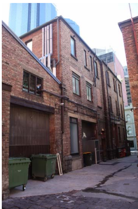
Figure 246 115-129 King Street, west wall to lane
