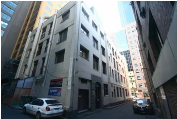
Figure 291 538-542 Little Collins Street- rear and side
