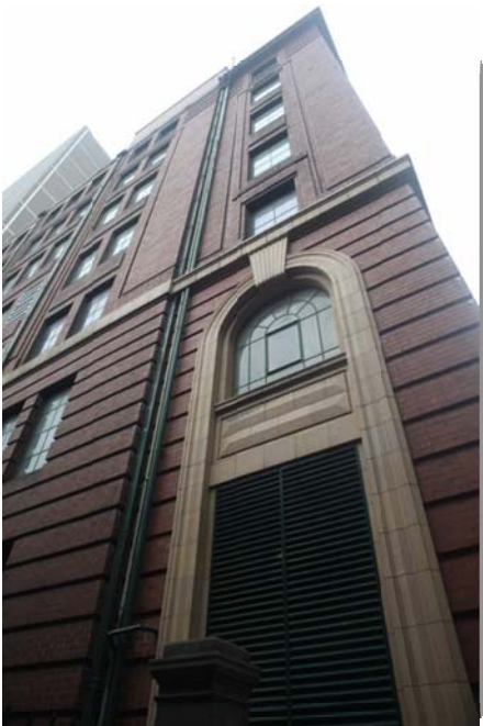
Figure 277 434-436 Little Bourke Street- precise façade detailing
