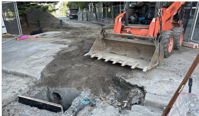
Works underway at the corner of Queensberry and Peel streets
