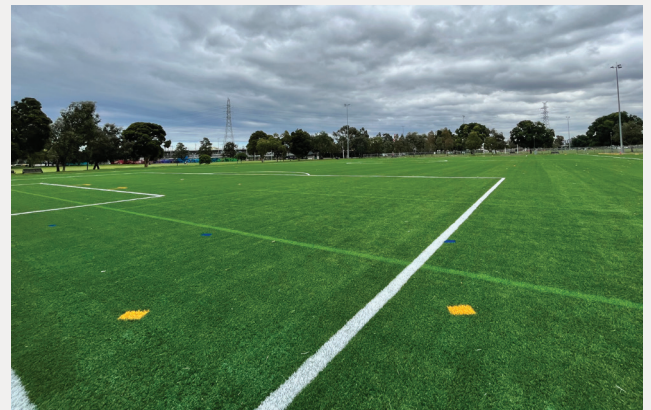
The resurfaced synthetic oval featuring new line markings
