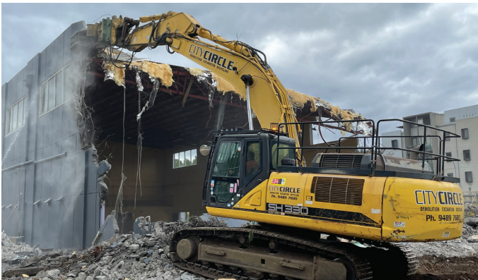
Demolition of the sports court is underway
