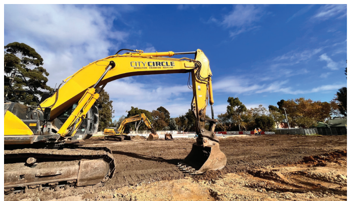
Demolition of the old centre is complete
